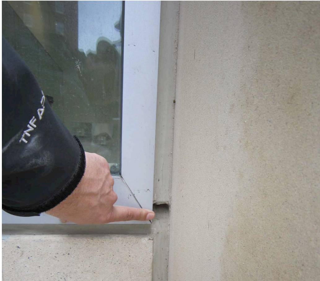
Figure 18: Weep hole in a drained two-stage joint
