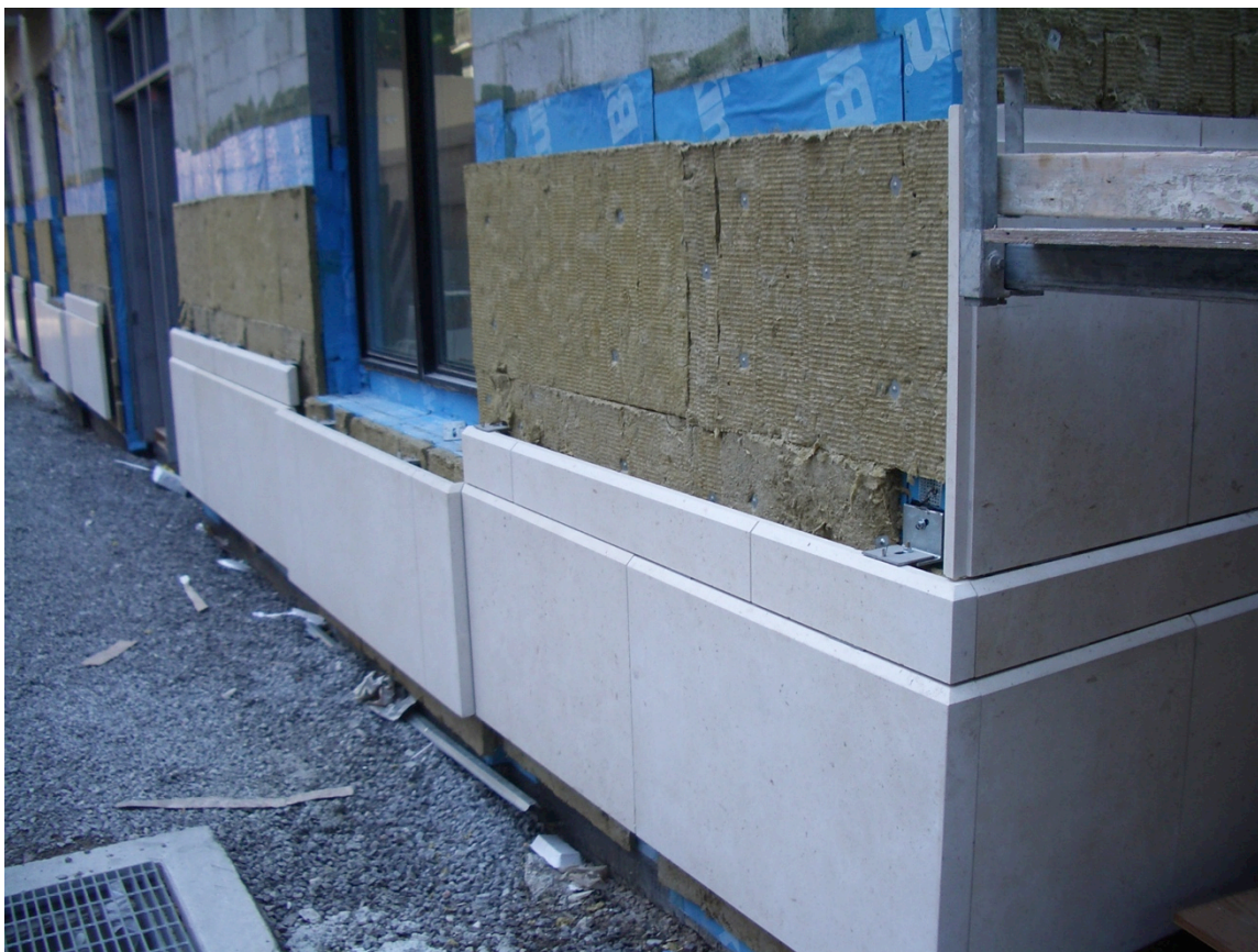
Figure 4: Small-format, handset precast installed as drained system
