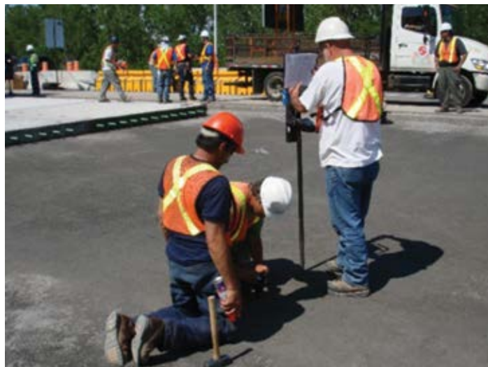
Figure 8.16. Survey crew using a robotically controlled total station to lay out panel points on a total replacement project. Source: The Fort Miller Co., Inc.
