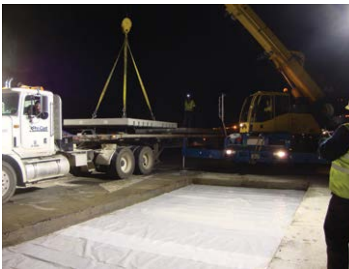
Figure 10.5. Panels arriving on trucks are easy to inspect for defects and flaws because all six sides of each panel are visible. Source: The Fort Miller Co., Inc.
