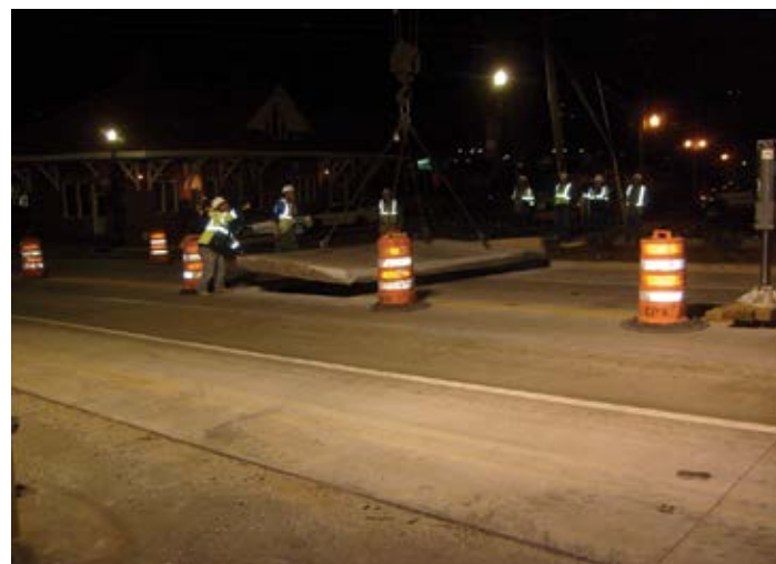
Figure 11.19. The damaged panel, less the concrete around the dowels, is removed. Source: The Fort Miller Co., Inc.
