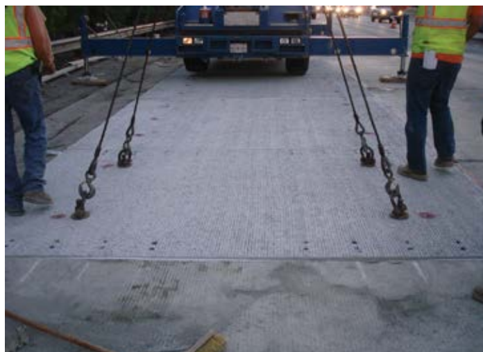
Figure 9.53. All the panels in the lane replacement repair area shown here were placed to leading end marks so the last panel being set precisely fits the space left by the previously placed transverse saw cut. Source: The Fort Miller Co., Inc.
