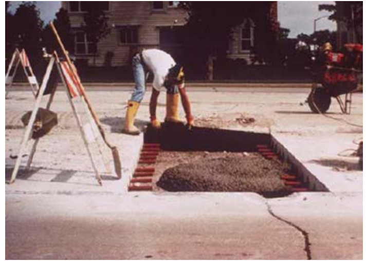
Figure 4.2. Use of isolation material between mismatched transverse joints. Source: National Concrete Pavement Technology Center
