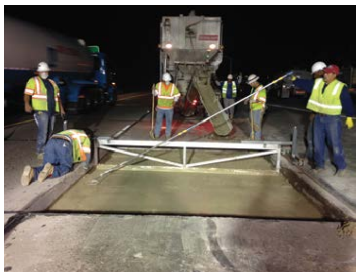
Figure 10.14. Two concrete finishers working behind four workers screeding newly placed lean concrete subbase. Source: The Fort Miller Co., Inc.
