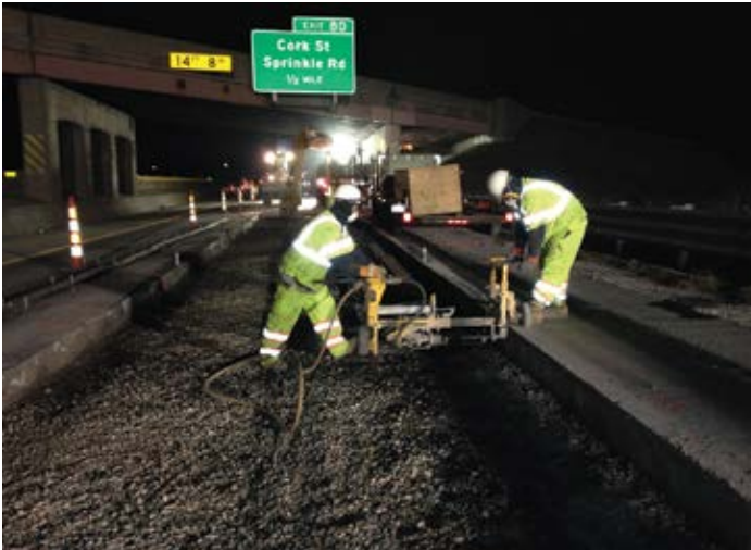
Figure 9.41. A single-bit air drill used for drilling tie bar holes at correct locations. Source: The Fort Miller Co., Inc.
