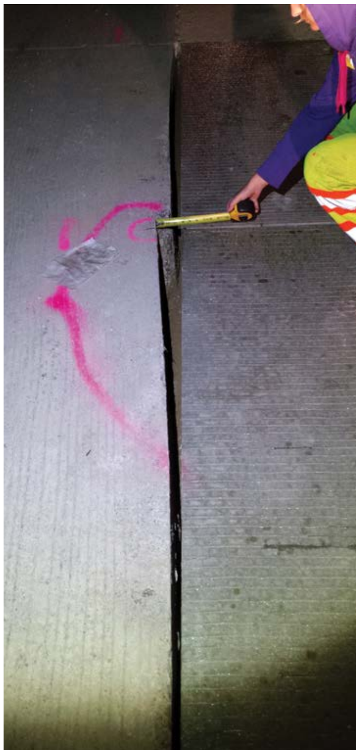
Figure 8.13. Example of an inaccurately sawed longitudinal joint. Source: The Fort Miller Co., Inc.
