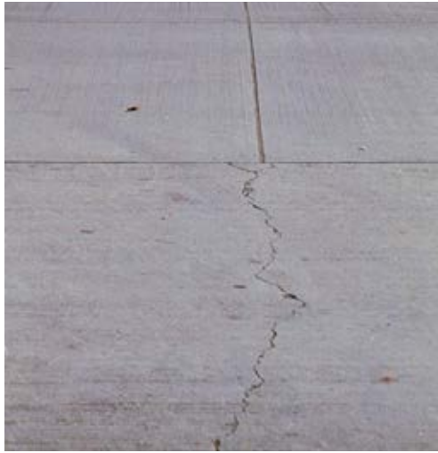
Figure 4.1. Transverse sympathy cracking due to mismatched transverse joints. Source: Jeff Uhlmeier, Washington State Department of Transportation
