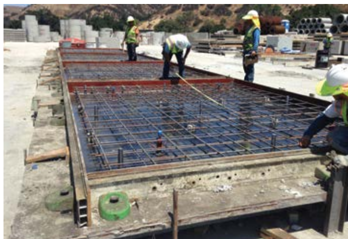
Figure 7.15. QC check of panel lengths just prior to concrete placement. Source: The Fort Miller Co., Inc.
