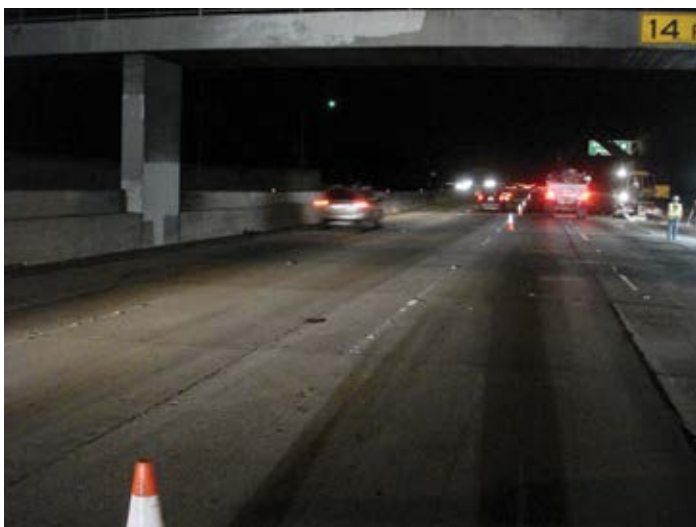
Figure 8.2. The work area on this five-lane California interstate project was three lanes wide, providing a safe, 12-foot-wide buffer zone. Source: The Fort Miller Co., Inc.
