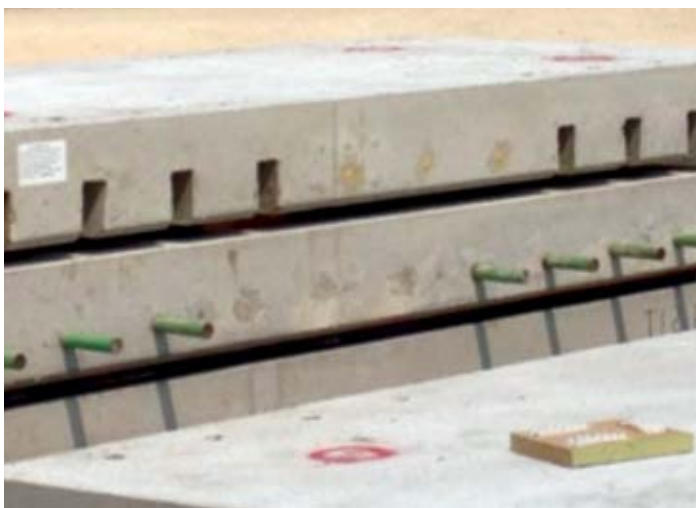
Figure 4.23. Precast panels with dowels translated vertically to provide thicker concrete over slots. Source: The Fort Miller Co., Inc.
