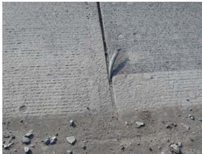
Figure 12.9. The bond between the silicone seal and concrete failed after approximately five years of service in this constant-width joint. Joint cleanliness problems are suspected. Source: The Fort Miller Co., Inc.
