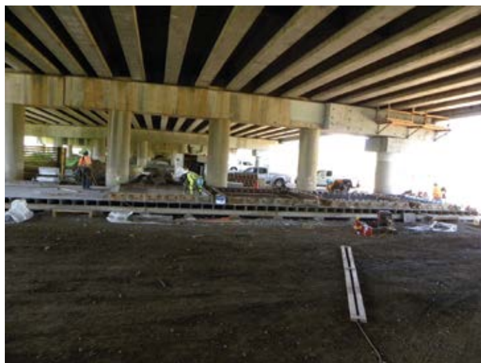
Figure 7.5. Plywood forms used at a contractor's on-site "precast yard." Source: Shiraz Tayabji, Applied Research Associates, Inc.
