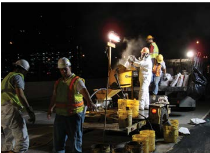
Figure 9.15. A grouting crew using a trailer-mounted batch-type mixer/pump. Source: The Fort Miller Co., Inc.
