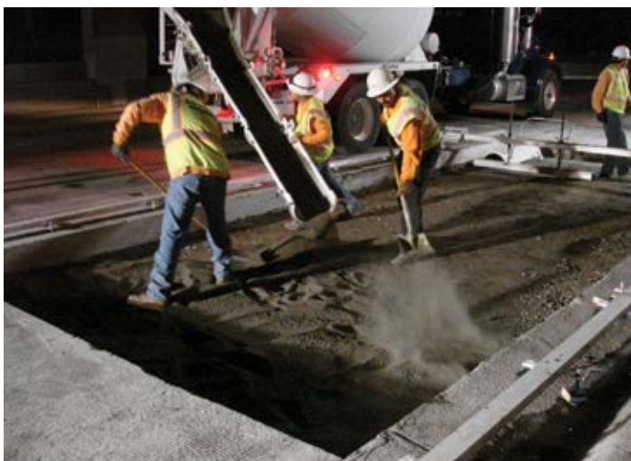
Figure 9.5. Cement-treated bedding material being discharged from a standard concrete truck. Source: The Fort Miller Co., Inc.
