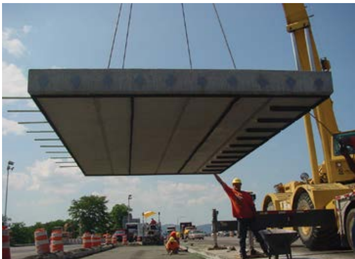
Figure 9.17. The bottom of a Super-Slab panel with built-in bedding grout distribution channels and black grout retention gaskets. Source: The Fort Miller Co., Inc.
