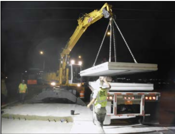
Figure 6.4. Rubber-tire excavator placing a 12-foot-wide-by-10-foot-long panel. The same equipment was also used to excavate and remove the existing pavement. Source: The Fort Miller Co., Inc.
