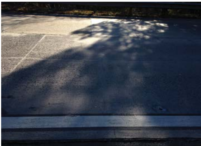
Figure 11.6. A transverse crack in the foreground lane lines up approximately with a joint at a cast-in-place concrete patch in the adjacent lane. Source: The Fort Miller Co., Inc.
