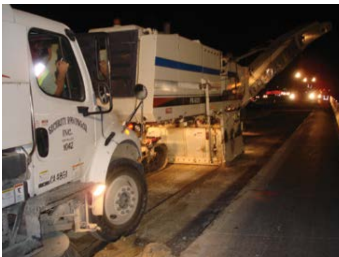
Figure 8.33. CTB removal with a large-scale milling machine, followed by a conventional "street sweeper" broom truck to ensure all milled material is removed. Source: The Fort Miller Co., Inc.
