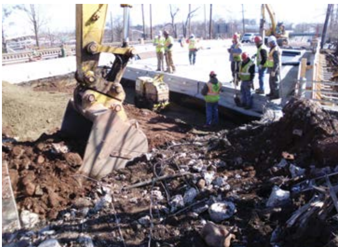
Figure 3.22. Replacement of bridge embankment material below approach slabs on the Route 46 Bridge in Clifton, N.J. Source: The Fort Miller Co., Inc.
