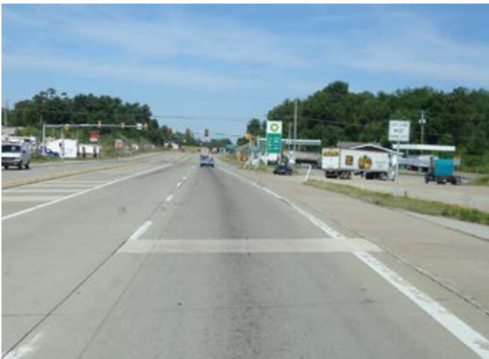
Figure 4.3. Concrete pavement with widened outside lane construction. Source: Pavement Engineering and Research Consultants, LLC
