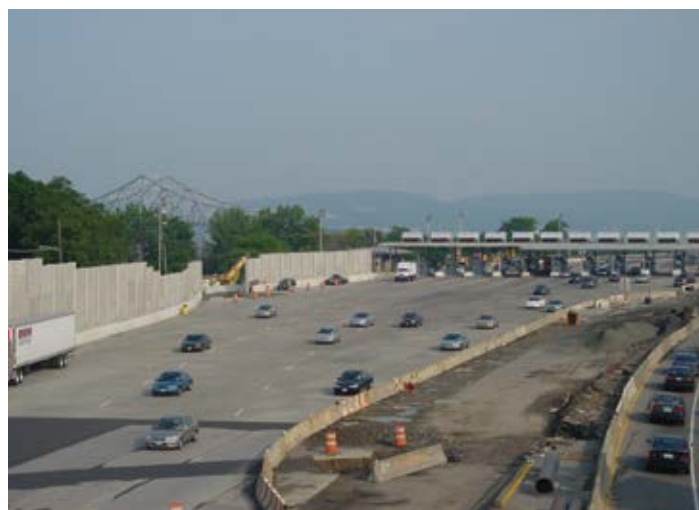
Figure 3.21. Tappan Zee Bridge toll plaza near Tarrytown, N.Y., after precast panel installation in 2002. Source: The Fort Miller Co., Inc.
