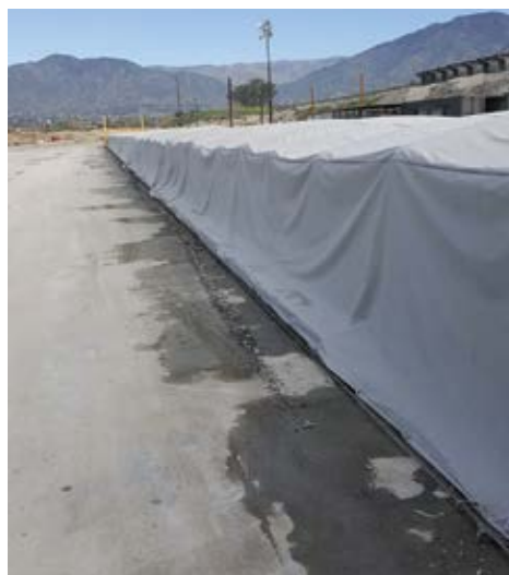
Figure 7.2. Long-line bed covered with insulated curing blankets to facilitate steam curing. Source: Pro-Cast Products
