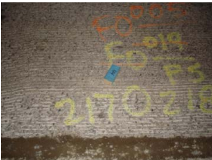
Figure 8.12. The black mark perpendicular to the edge of the pavement (dark gray) represents the leading end of panel 217. Source: The Fort Miller Co., Inc.
