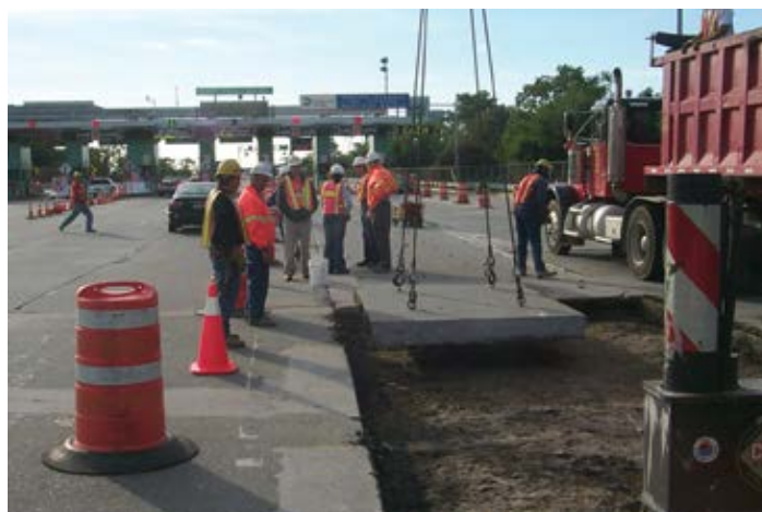
Figure 8.22. Slabs being removed using the lift-out method. Notice the spalls on the edge of the remaining pavement on the left caused by the lifting operation. Source: The Fort Miller Co., Inc.
