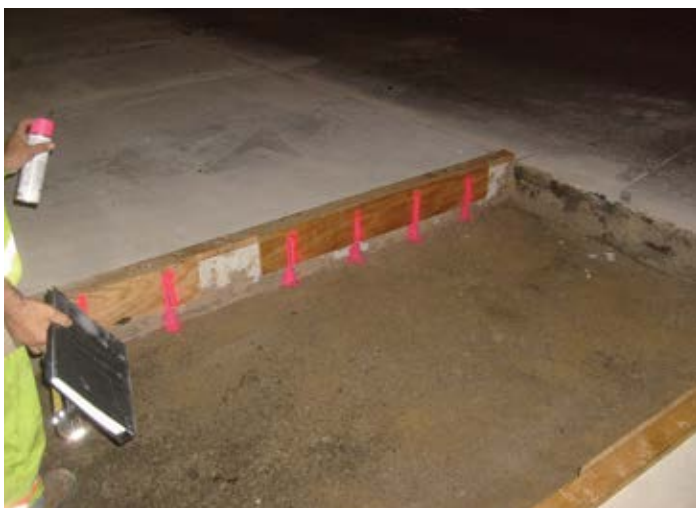
Figure 9.25. The template seen here consists of pre-drilled plywood supported by an attached 2-inch-by-4-inch horizontal member. Source: The Fort Miller Co., Inc.
