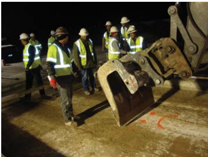
Figure 8.31. Trimming isolated high spots in CTB (red marks) with an excavator bucket. Source: The Fort Miller Co., Inc.
