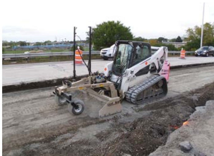
Figure 9.4. A laser-equipped skid-steer and grading box using a digital surface model for grade control. Source: The Fort Miller Co., Inc.
