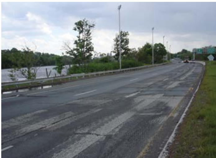
Figure 3.30. Milled composite pavement on Route 21 in New Jersey. Source: The Fort Miller Co., Inc.
