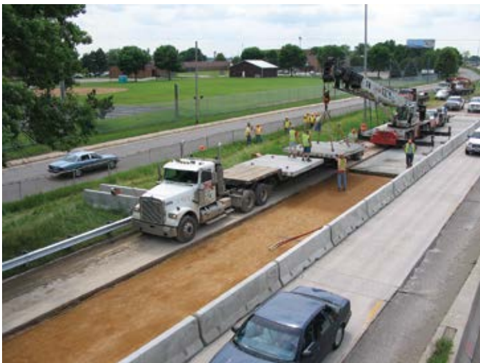
Figure 2.2. Example use of two lanes to perform repairs in a single lane. Source: Wieser Concrete Products
