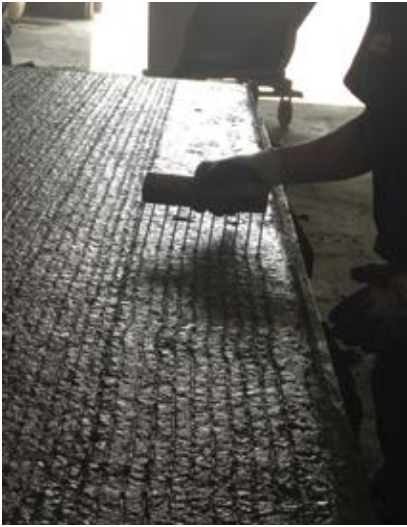
Figure 7.24. Use of a narrow, custom-width rake to texture a narrow strip at the edge of a panel. Source: The Fort Miller Co., Inc.
