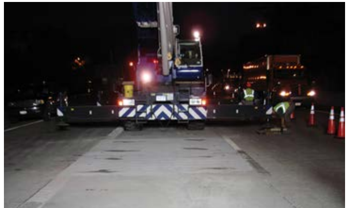
Figure 8.1. Men working approximately 8 feet away from live traffic, separated only by traffic cones. Source: The Fort Miller Co., Inc.
