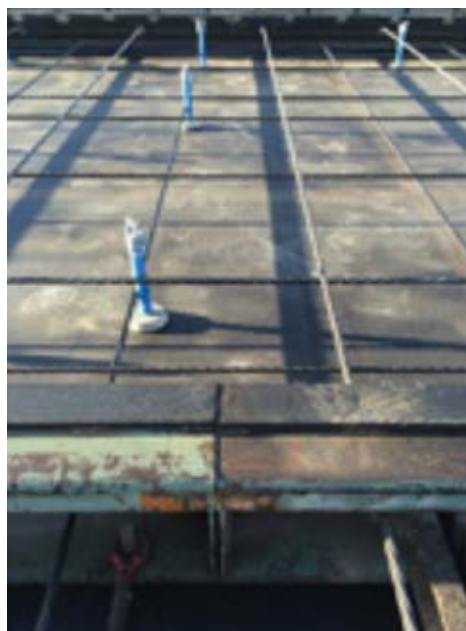
Figure 7.17. An example of prestressing strand used in two directions. Source: Con-Fab California, LLC
