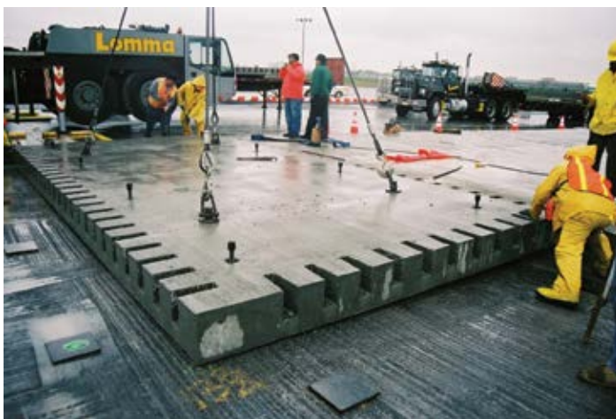
Figure 3.31. Installation of precast taxiway panels at LaGuardia Airport. Source: Shiraz Tayabji, ARA Inc.
