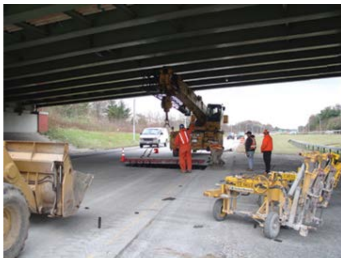
Figure 2.5. Example use of an excavator placing PCP panels beneath an overpass. Traffic is maintained on the lane to the right of the excavator. Source: The Fort Miller Co., Inc.
