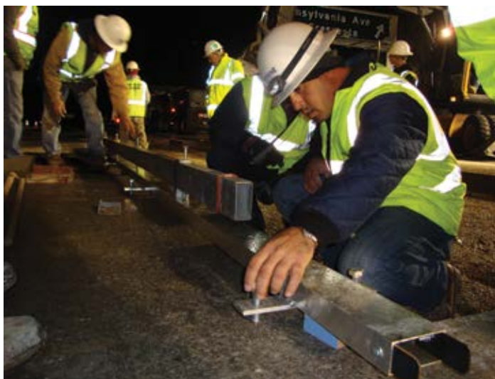
Figure 10.7. A grading crew checks and adjusts screed rails to ensure an accurate grading frame of reference. Source: The Fort Miller Co., Inc.
