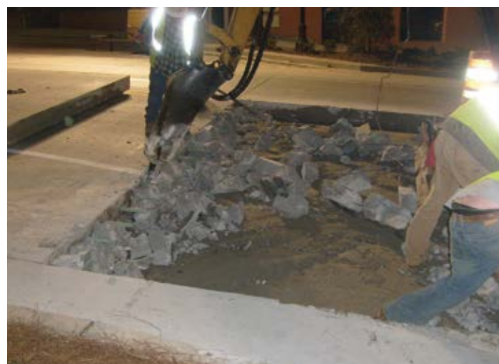
Figure 11.20. A small hoe ram removing concrete around dowels that are to remain in place. Source: The Fort Miller Co., Inc.
