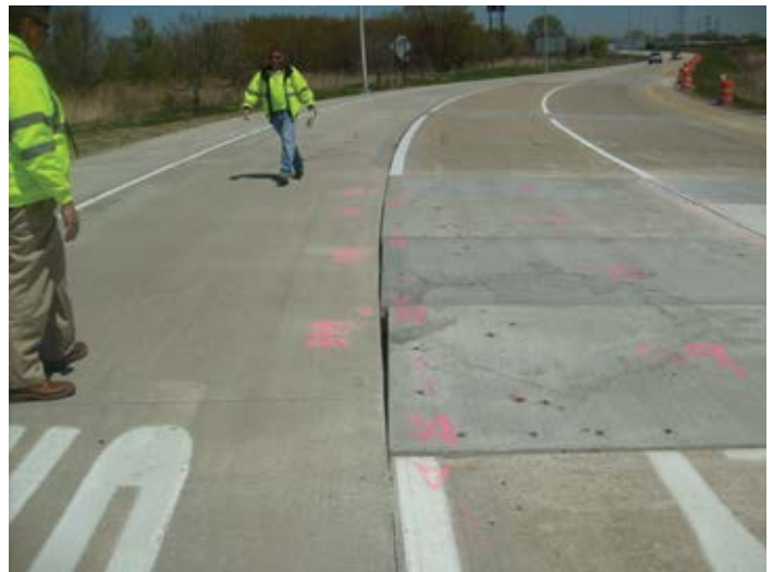
Figure 8.11. Example of a "saw-tooth" longitudinal joint created because the end cut, seen in the foreground, was not laid out and cut radially to the horizontal curve. Source: The Fort Miller Co., Inc.
