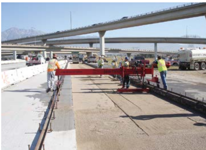
Figure 9.3. A larger, hand-operated grader controlled by pre-set grade rails set to specific elevations. Source: The Fort Miller Co., Inc.
