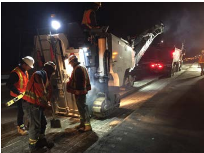
Figure 13.15. A 1.2-meter-wide milling machine makes a full-depth pass. Source: The Fort Miller Co., Inc.
