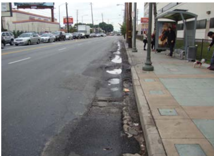
Figure 3.24. Bus pad pavement prior to replacement in North Hollywood, Calif. Source: The Fort Miller Co., Inc.
