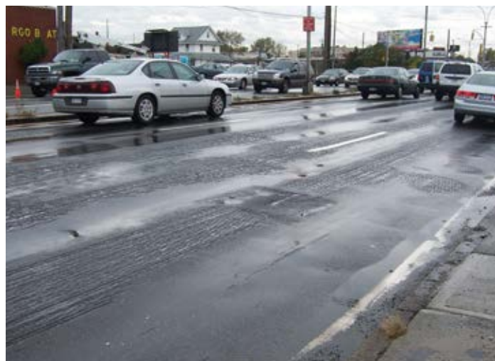
Figure 3.17. Heavily rutted asphalt pavement on Rockaway Boulevard in Queens, N.Y. Source: The Fort Miller Co., Inc.
