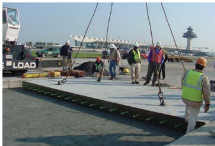
Figure 3.32. Installation of precast taxiway panels at Dulles International Airport. Source: The Fort Miller Co., Inc.
