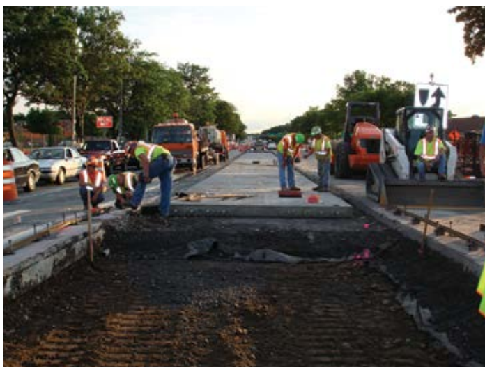
Figure 2.12. Undercutting foundation prior to placing PCP panels on Route 7 near Rotterdam, N.Y. Source: The Fort Miller Co., Inc
