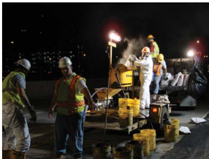
Figure 10.18. On-the-job training of a grout crew. Source: The Fort Miller Co., Inc.
