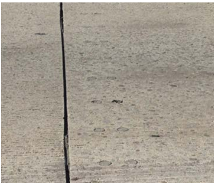
Figure 12.10. Grout in some dowel grout ports may have de-bonded here, potentially allowing water to penetrate to the dowel bar level. Source: The Fort Miller Co., Inc.
