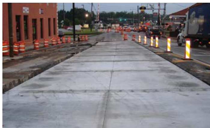
Figure 11.25. Severe cross-slope and vertical profile grade changes at the far end of new panels. Source: The Fort Miller Co., Inc.
