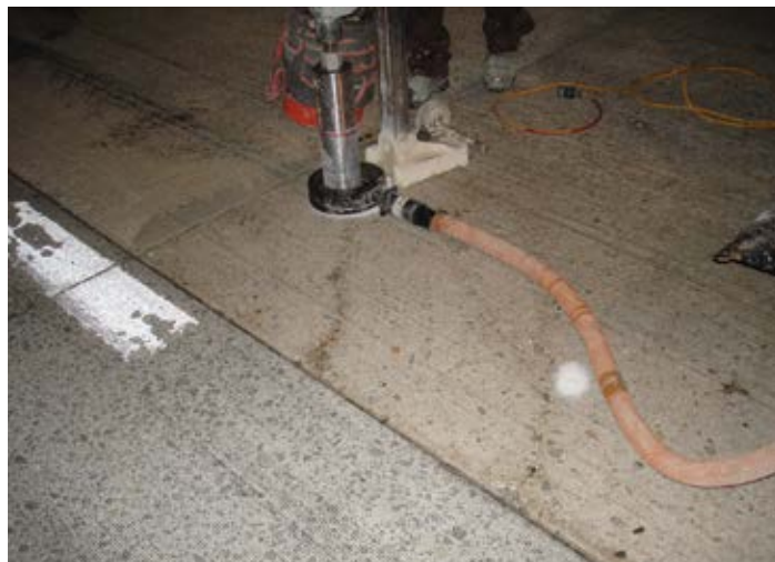
Figure 11.7. This diagonal crack – visible because it is wet – emanated from a bottom slot directly under the core drill. The crack was likely caused by inadequate corner support resulting from improper grading and/or installation of bedding grout. Source: The Fort Miller Co., Inc.
