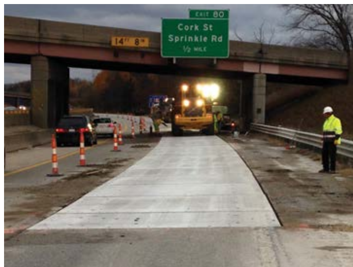
Figure 8.5. Traffic being diverted to the left shoulder, leaving a partial lane, a full lane and the shoulder on the right as a safe working area. Source: The Fort Miller Co., Inc.
