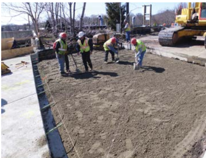
Figure 10.15. A grading crew using string lines (foreground) to check the rough grade of bedding material. Source: The Fort Miller Co., Inc.
