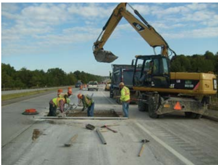
Figure 8.26. The versatile rubber-tire excavator can be used for removal, rough grading and placement of new panels up to 10 feet by 12 feet. Source: The Fort Miller Co., Inc.
