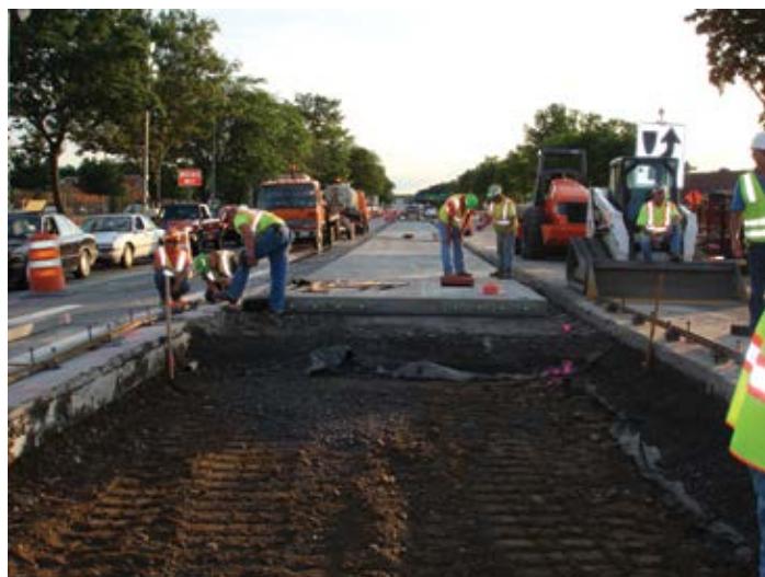
Figure 8.27. An example of undercutting 1 foot prior to replacement with geo-fabric, new subbase material and JPrCP panels. Source: The Fort Miller Co., Inc.
