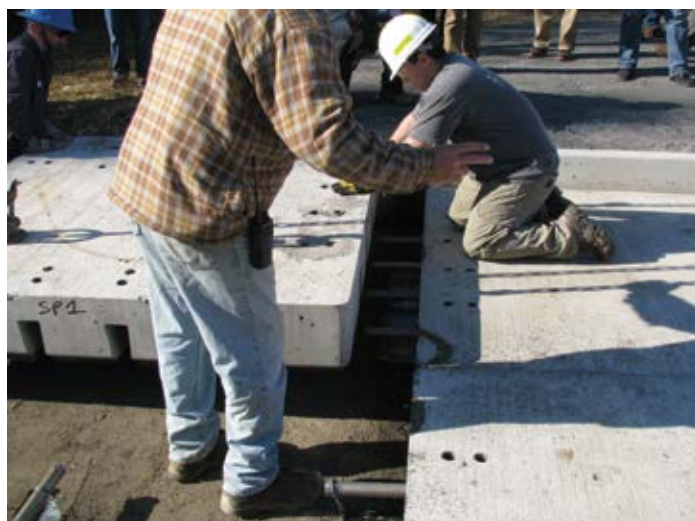
Figure 13.12. Super-Paver unit being installed over Super-Dowels in adjacent units. Source: The Fort Miller Co., Inc.
