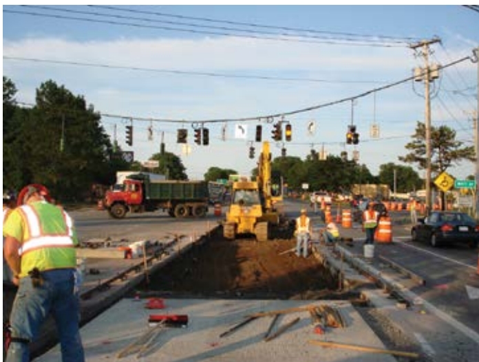
Figure 2.4. Sources of potential vertical clearance issues during installation. Source: The Fort Miller Co., Inc.
