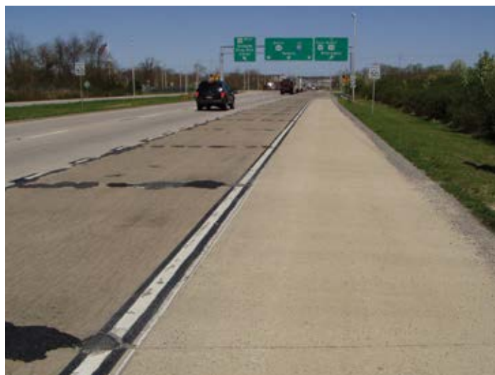
Figure 2.9. Joint failure on concrete pavement. Source: The Transtec Group, Inc.
