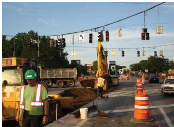
Figure 3.15. Street view of the pavement replacement operations at the intersection of Route 7 and Nott Street in Rotterdam, N.Y. Source: The Fort Miller Co., Inc.
