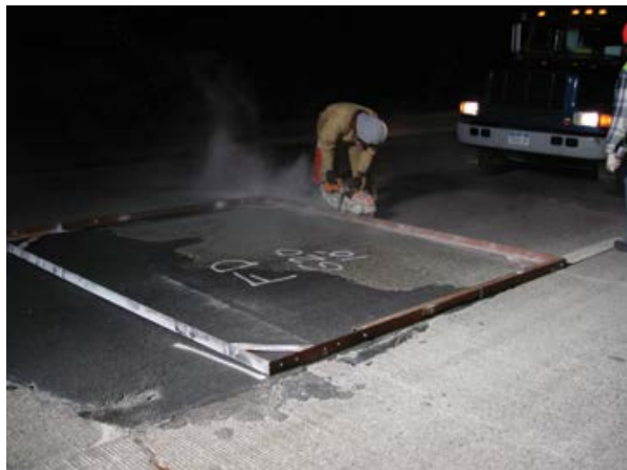
Figure 8.8. An example of a contractor-designed steel template being used to lay out saw cut lines for a single panel. Source: The Fort Miller Co., Inc.
