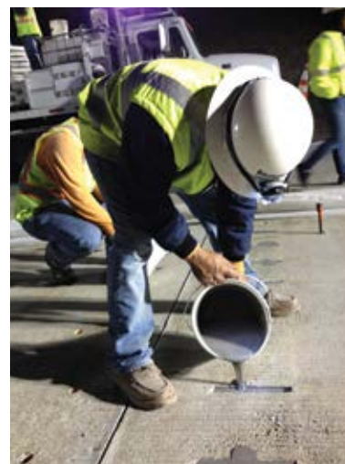
Figure 9.32. Latex grout being poured into the narrow top slot of the Barra Glide system. Source: Performance Plus Products, LLC
