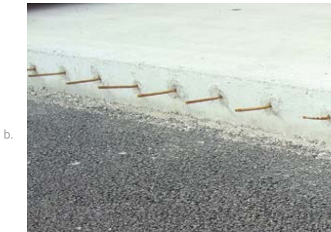
Figure 4.17. Schematic of a tied longitudinal construction joint with optional keyway and photo of tie bars along longitudinal joint.
