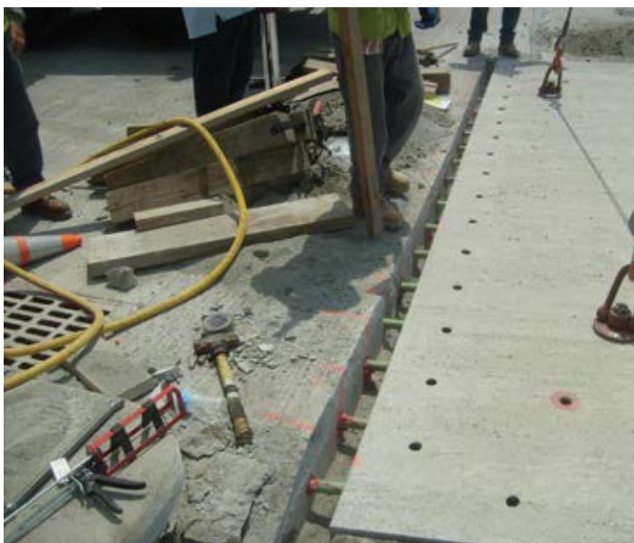
Figure 12.5. This excessively wide transverse joint resulted from cutting the existing pavement on the left at the incorrect location. Source: The Fort Miller Co., Inc.
