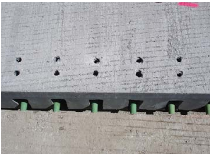
Figure 9.23. A Super-Slab panel being lowered over the dowels of a previously placed panel. Source: The Fort Miller Co., Inc.
