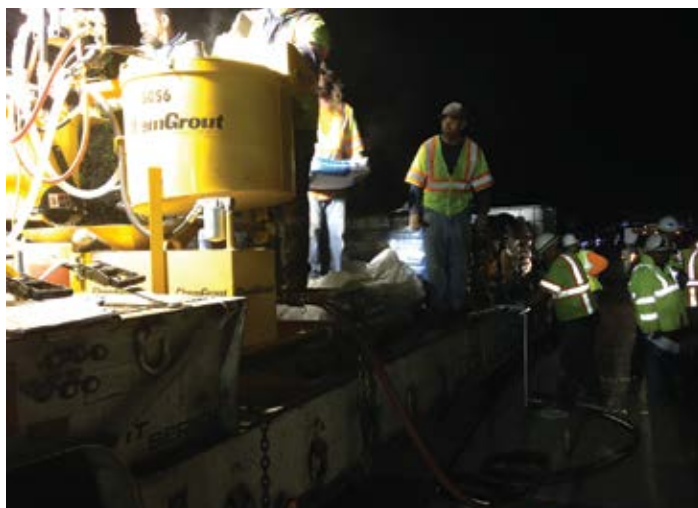
Figure 9.19. A dual-drum, high-capacity mixer/pump mounted on a service trailer with an adequate supply of grout and water and a safe working space. Source: The Fort Miller Co., Inc.
