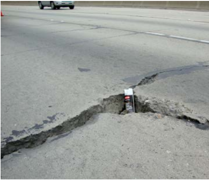
Figure 1.1. Photo of deteriorated concrete pavement. Source: Performance Plus Products, LLC
