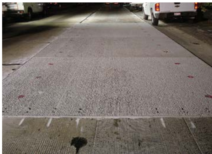
Figure 11.27. These panels, finished at the precast plant with a burlap-drag-and-raked finish, did not require diamond grinding. Friction requirements were met during panel fabrication and smoothness requirements were met during panel placement. Source: The Fort Miller Co., Inc.
