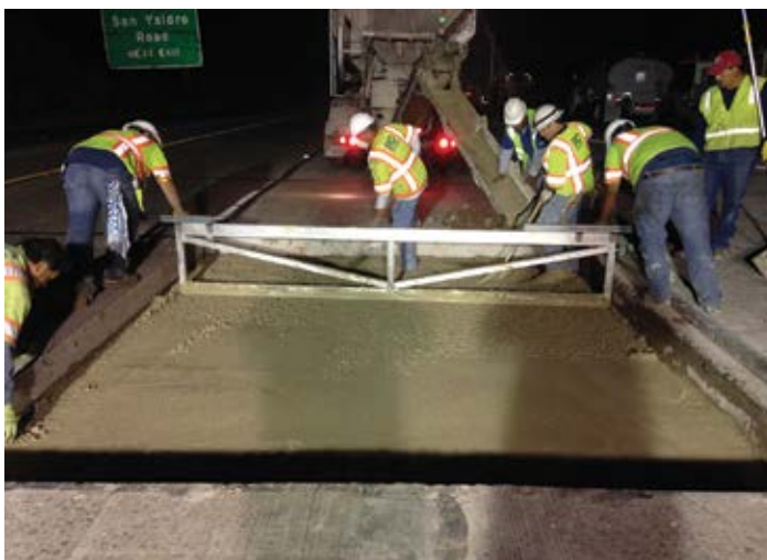
Figure 9.7. A wheel-mounted concrete screed using a pre-set rail on one side of the hole and the existing pavement on the other as a grade reference. Source: The Fort Miller Co., Inc.
