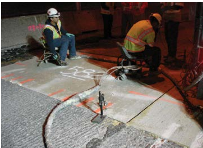
Figure 9.11. Two workers, each equipped with a urethane injector tip, installing foam to the underside of the panels through foam ports. Source: The Fort Miller Co., Inc.
