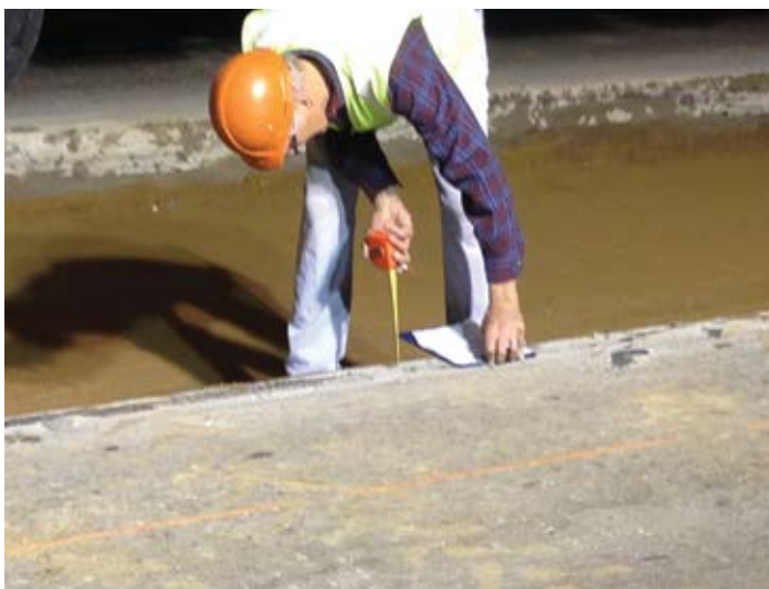
Figure 10.10. A DOT inspector checks the finished elevation and grading of the subbase. Source: The Fort Miller Co., Inc.
