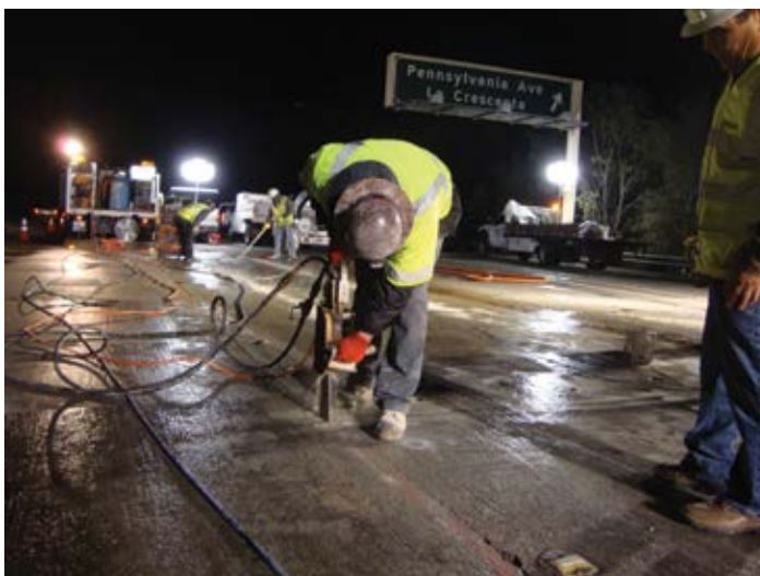
Figure 8.20. A concrete chainsaw equipped with diamond teeth is used to finish a full-depth saw cut without overcutting into the adjacent panel. Source: The Fort Miller Co., Inc.
