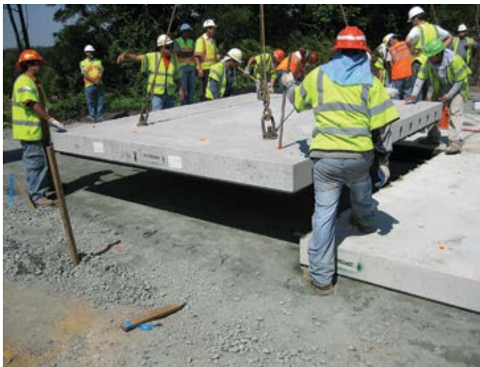
Figure 10.1. State DOT engineers witness the installation of a precast panel at a system trial installation. Source: The Fort Miller Co., Inc.
