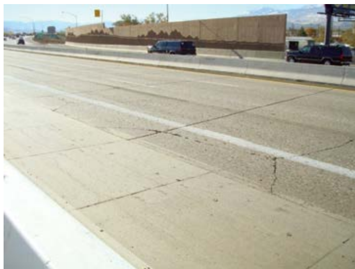
Figure 2.13. Precast panels placed next to cracked panels on Interstate 395 near Reno, Nev. Source: The Fort Miller Co., Inc.
