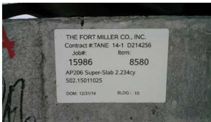
Figure 7.28. Example panel label showing all the information needed for identification purposes. Source: The Fort Miller Co., Inc.
