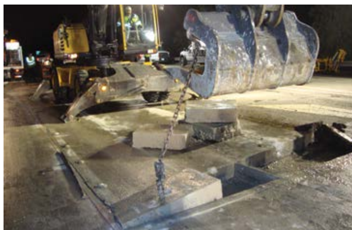
Figure 8.25. Excavator removal using a slab crab bucket, showing little disturbance of the underlying subbase. Source: The Fort Miller Co., Inc.
