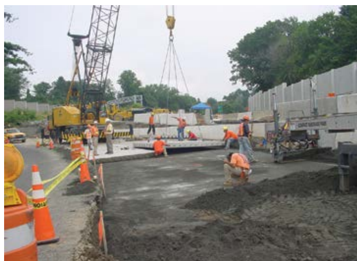
Figure 9.49 Because equal-length picking cables were used over a sloped surface, PCP panels on this project had to be placed numerous times to bring joint widths within specified tolerances. Source: The Fort Miller Co., Inc.
