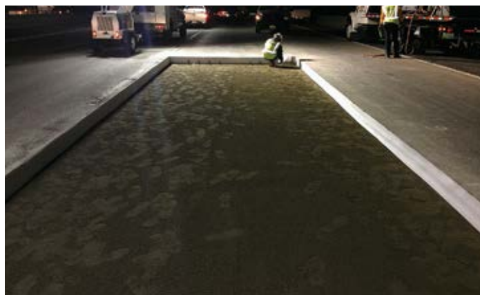
Figure 11.29. 1/2-inch-thick white isolation foam attached to the longitudinal edge of the existing pavement. Source: The Fort Miller Co., Inc.
