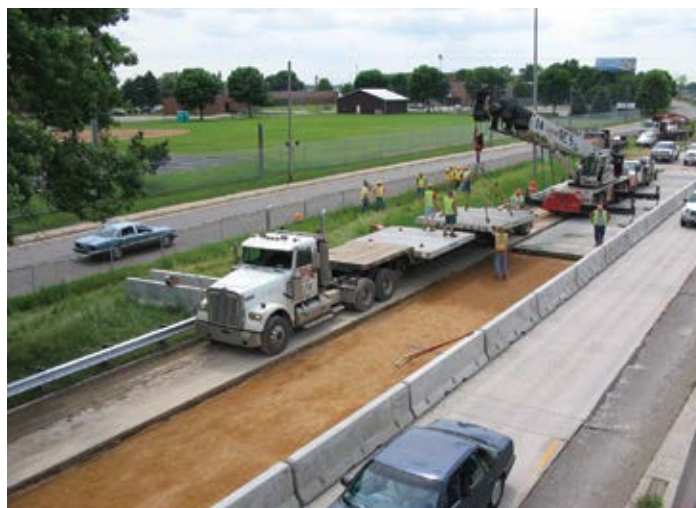
Figure 9.46. A 65-ton capacity hydraulic crane picking panels from a truck positioned in front of, rather than alongside, the crane. Source: Wieser Concrete Products
