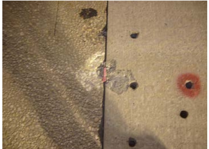
Figure 11.2. Transverse joint spalls in both the existing pavement and the new precast panel in this photo resulted from the red shim pad – placed to keep adjacent panels from hitting each other – being placed too close to the surface. Source: The Fort Miller Co., Inc.
