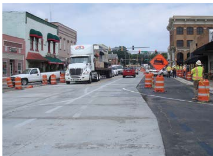
Figure 3.18. New precast panels on Broad Street in Winder, Ga. Source: The Fort Miller Co., Inc.
