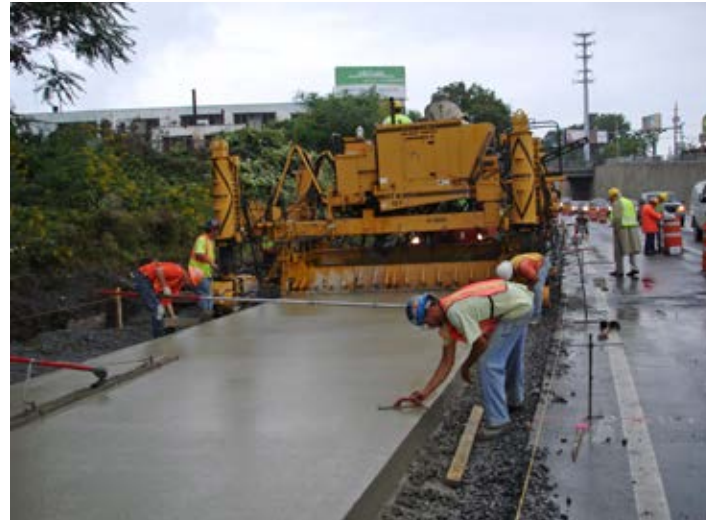
Figure 1.4. Plastic concrete extruded to correct grade and cross-slope behind slip-form paver. Source: The Fort Miller Co., Inc.
