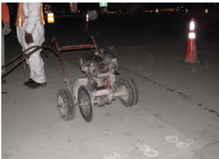
Figure 11.33. A joint cutting saw equipped with a stack of blades equal to the desired joint width. Source: The Fort Miller Co., Inc.
