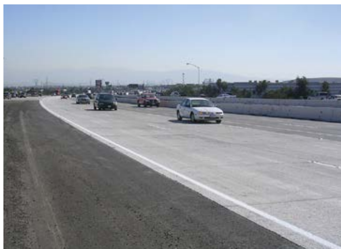
Figure 3.9. Lane replacement of a curved portion of Interstate 15 near Ontario, Calif., using JPrCP. Source: The Fort Miller Co., Inc.
