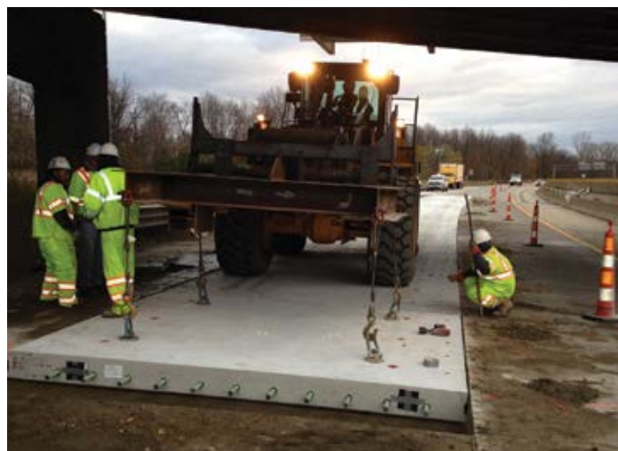
Figure 9.51. A large loader carrying and placing a PCP panel under an interstate overpass. Source: The Fort Miller Co., Inc.
