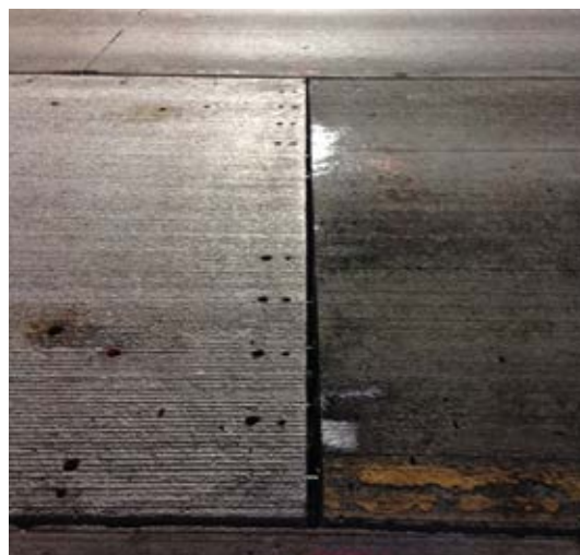
Figure 11.12. The transverse joint seen here varies in width from about 1/2 inch on the far end to approximately 2 inches on the near end because of incorrect saw cutting of the existing pavement. Source: The Fort Miller Co., Inc.
