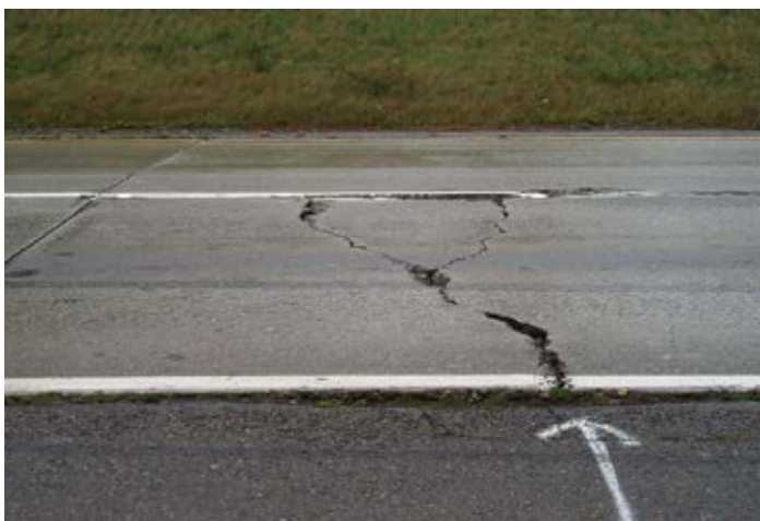
Figure 2.8. Deteriorating transverse crack on concrete pavement. Source: pavementinteractive.org
