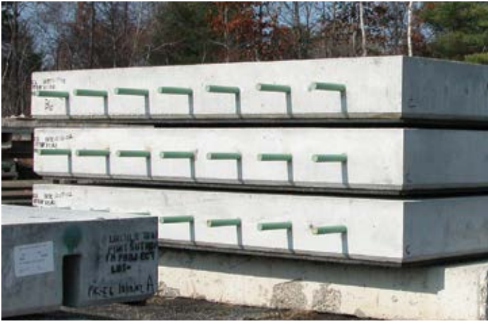
Figure 4.16. Half-embedded dowels in a JPrCP panel. Source: The Fort Miller Co., Inc.
