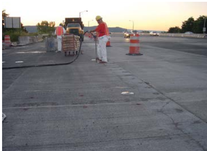
Figure 9.18. A worker pumping bedding grout into one end of a distribution channel until it comes out the other, a technique that verifies bedding grout has flowed under pressure for the entire length of the channel, indicating full distribution of grout under the panel. Source: The Fort Miller Co., Inc.
