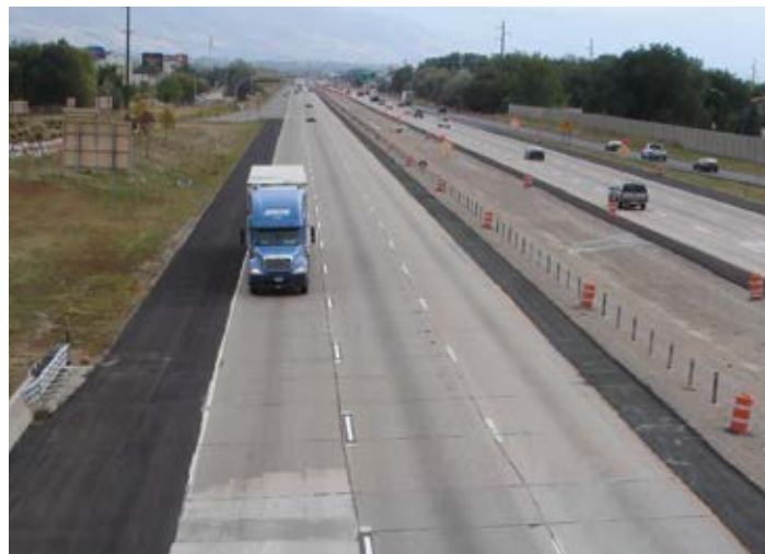
Figure 11.24. The existing pavement on both the approach and leave ends of this panel was ground because the precast panel was placed too low. Source: The Fort Miller Co., Inc.
