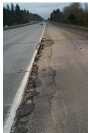
Figure 2.11: Joint and crack faulting with severe pumping, indicating drainage and erosion problems. Source: PavementInteractive.com
