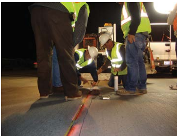
Figure 10.6. A contractor's crew checks saw cut layout lines prior to sawing. Source: The Fort Miller Co., Inc.
