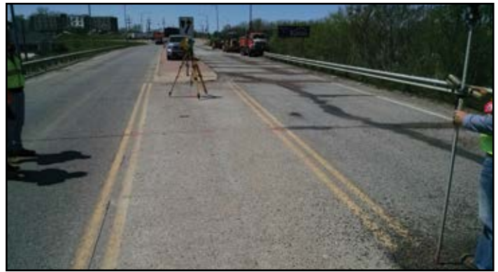
Figure 6.6. Collection of existing pavement data using a robotically controlled total station. Source: The Fort Miller Co., Inc.
