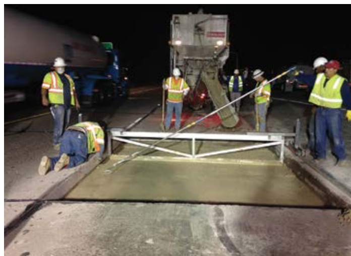
Figure 9.8. Masons finishing new lean concrete subbase behind the concrete screed. Source: The Fort Miller Co., Inc.
