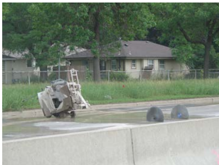
Figure 8.21. Saw blades bound up by slab expansion in hot weather. Source: The Fort Miller Co., Inc.
