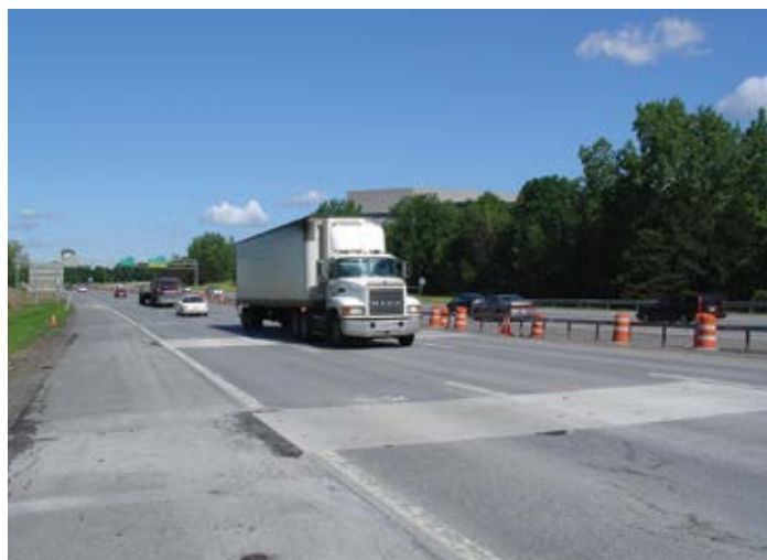
Figure 3.3. Six-foot-long, full lane-width joint repair panels in adjacent lanes. Source: The Fort Miller Co., Inc.
