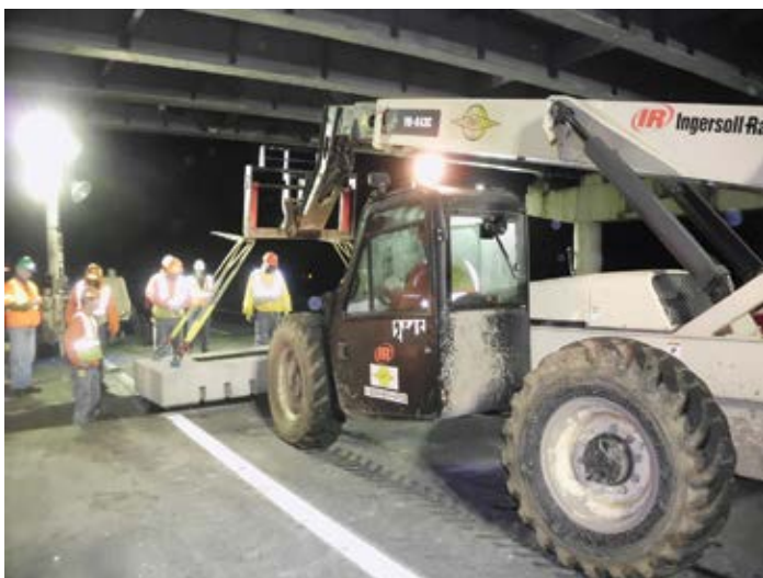
Figure 2.6. Example use of a fork truck to install PCP panels beneath an overpass. Source: The Fort Miller Co., Inc.
