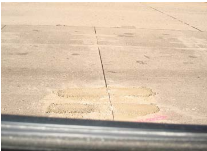
Figure 11.5. The original dowels in the top slots seen in the foreground were sawed out and replaced with new, full-length dowels and the slot was backfilled with polyester concrete. Source: The Fort Miller Co., Inc.
