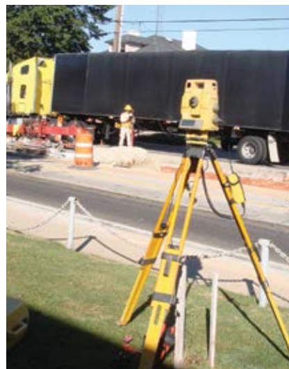
Figure 10.11. A surveyor establishes panel points and grades for a continuous PCP. Source: The Fort Miller Co., Inc.
