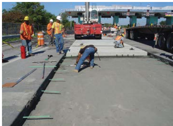
Figure 9.48. Both sets of outriggers on this hydraulic crane are positioned on existing pavement. Source: The Fort Miller Co., Inc.
