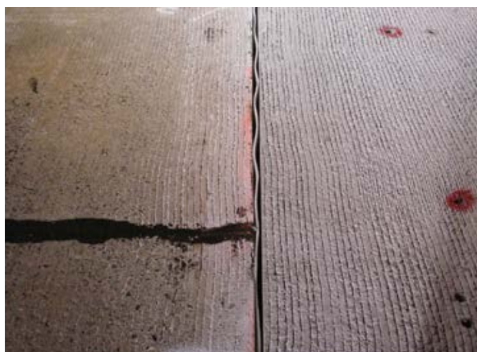
Figure 11.30. The isolation foam in this longitudinal joint does not completely fill the joint. Source: The Fort Miller Co., Inc.
