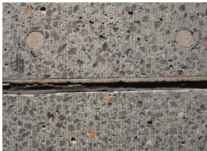
Figure 11.34. The sealant reservoir in this over-width joint was incorrectly cut with a 1/2-inch-wide blade. The remaining grout has already de-bonded from the existing pavement and is ready to fall out of the joint. Source: The Fort Miller Co., Inc.
