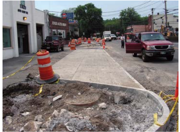
Figure 13.20. Non-planar, specially shaped precast panels were manufactured to meet the adjacent granite curb and pronounced surface contours while providing continuous commercial access. Source: The Fort Miller Co., Inc.
