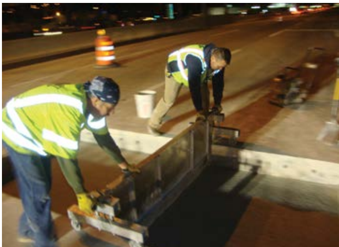
Figure 9.1. Screeding device using adjacent existing pavement as the frame of grade reference. Source: R.W. Dunteman
