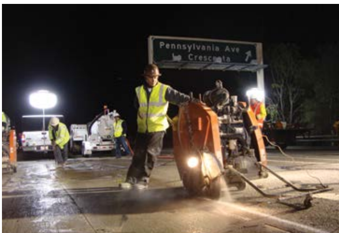
Figure 10.12. A sawing crew consisting of two saw operators and one slurry cleanup man. Source: The Fort Miller Co., Inc.
