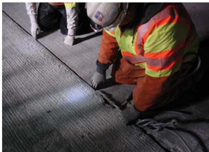
Figure 11.32. Small-diameter backer rod being braided together to fill a variable-width longitudinal joint prior to sealing. Source: The Fort Miller Co., Inc.
