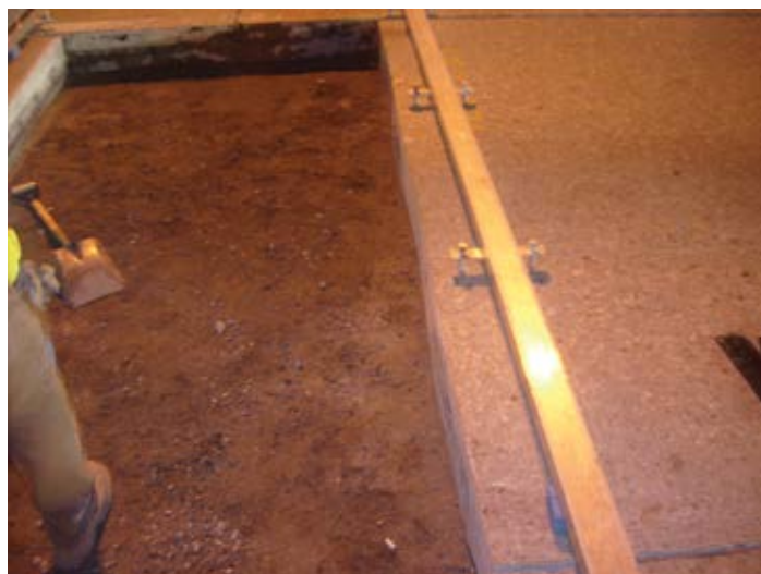
Figure 8.18. An undulating vertical saw cut made with a blade that was likely too flexible for the pavement. Source: The Fort Miller Co., Inc.
