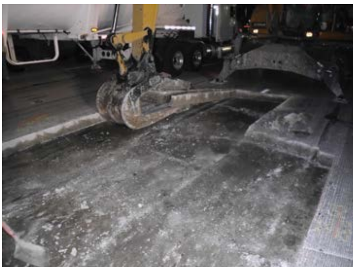
Figure 8.23. Removal of existing pavement using the excavator method with a slab crab. Source: The Fort Miller Co., Inc.
