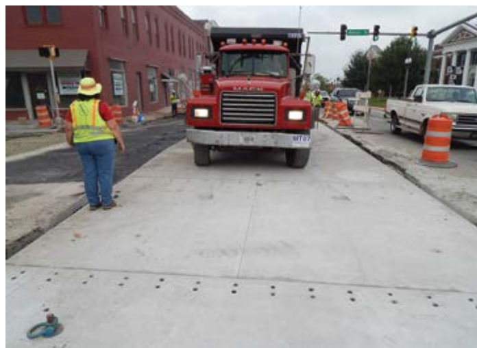
Figure 4.5. Installation of wide panels (travel lane plus shoulder) in Winder, Ga. Source: The Fort Miller Co., Inc.
