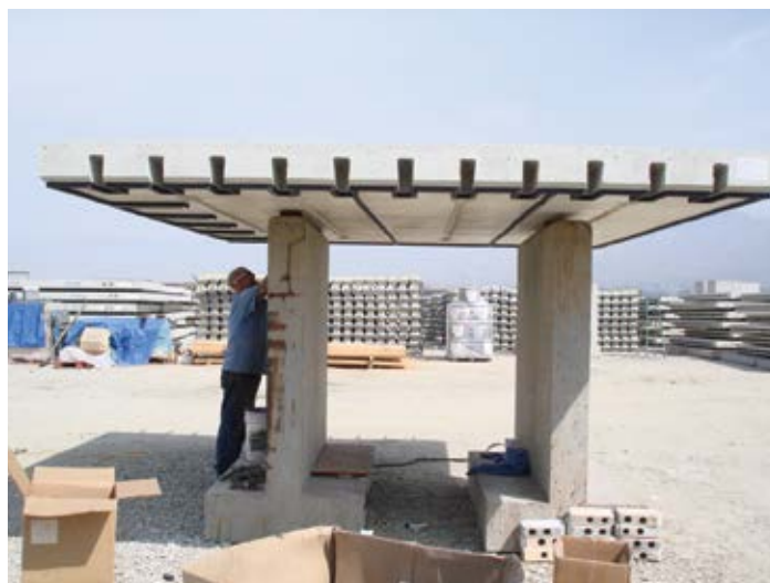
Figure 7.27. Applying foam gaskets to bottom of Super-Slab panels that have been placed on high stands. Source: The Fort Miller Co., Inc.
