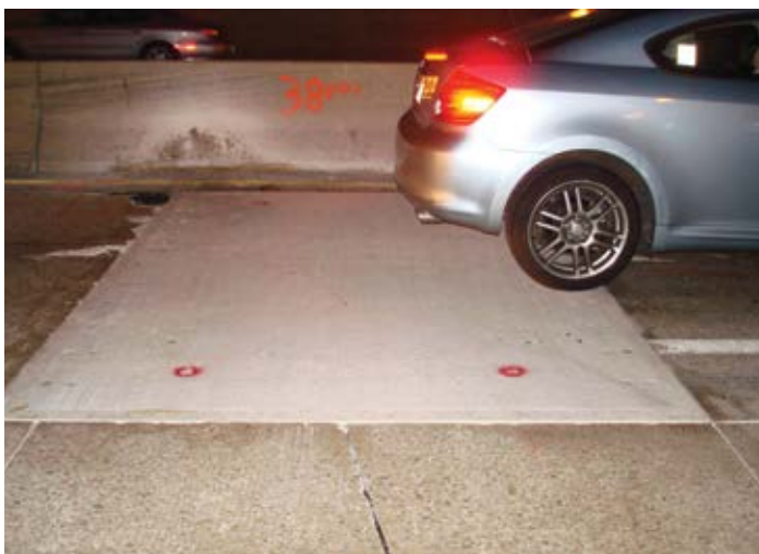
Figure 3.2. Eight-foot-long, full lane-width joint repair panel placed in a single lane. Source: The Fort Miller Co., Inc.
