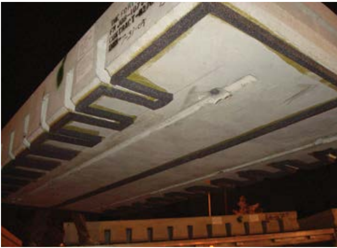
Figure 4.10. Proprietary grout distribution channels and gasket material on a Super-Slab JPrCP panel. Source: Pavement Engineering and Research Consultants, LLC
