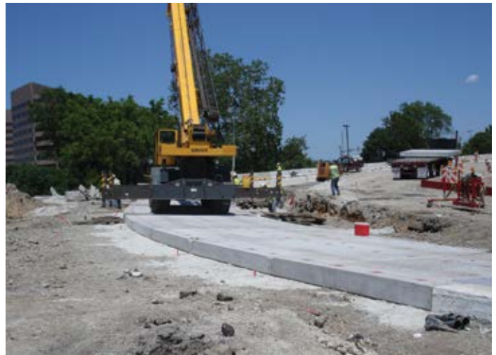
Figure 3.10. “Tight-radius” single-lane ramp in Chicago, Ill., that was replaced during a single weekend closure. Source: The Fort Miller Co., Inc.
