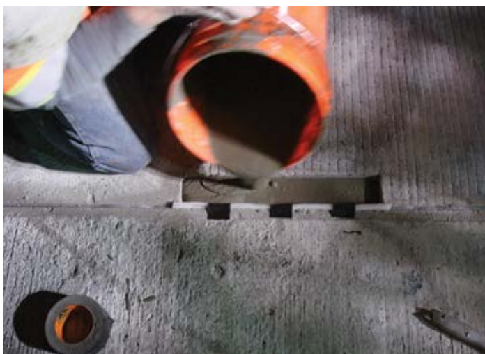
Figure 11.3. Two layers of foam (with black tape adhered to the near panel) were used along this transverse joint to retain the joint reservoir for the joint sealing material while repair material was installed. Source: The Fort Miller Co., Inc.
