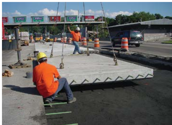
Figure 4.9. Placement of grade-supported precast panel for overnight use prior to installation of bedding grout at Tappan Zee Toll Plaza in New York. Source: The Fort Miller Co., Inc.
