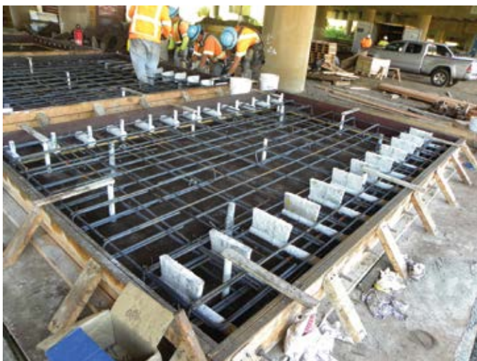
Figure 7.5. Plywood forms used at a contractor's on-site "precast yard." Source: Shiraz Tayabji, Applied Research Associates, Inc.
