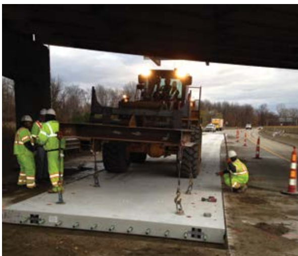
Figure 3.26. Placement of repair panels beneath an overpass on westbound Interstate 94 (Business Loop) near Kalamazoo, Mich. Source: The Fort Miller Co., Inc.
