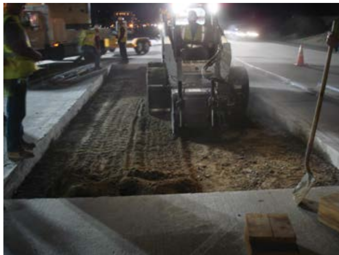
Figure 8.32. A skid-steer-mounted milling head trimming a large area of CTB. Source: The Fort Miller Co., Inc.
