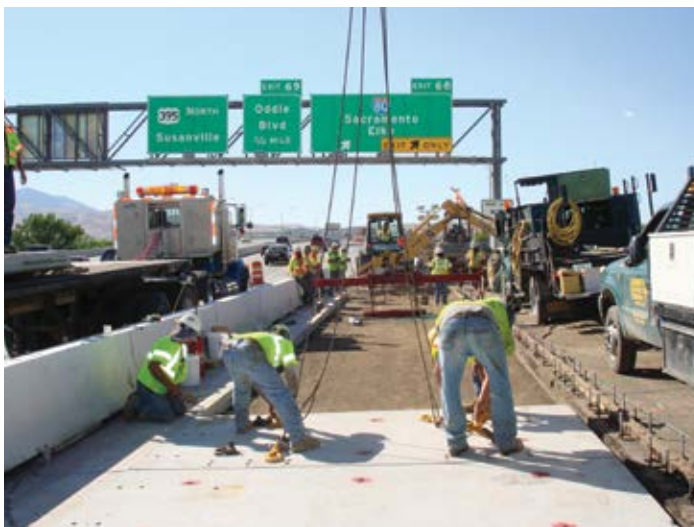
Figure 8.4. The work area allowed on this three-lane interstate was restricted to one lane, a small portion of the adjacent lane and the shoulder on the right. Source: The Fort Miller Co., Inc.
