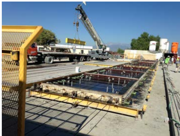
Figure 1.9. Photo of JPrCP fabrication in a prestressing bed. Source: Pro-Cast Products
