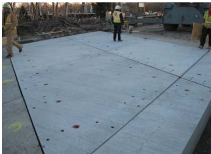
Figure 3.23. New precast concrete bridge approach panels at the Route 46 Bridge in Clifton, N.J. Source: The Fort Miller Co., Inc.
