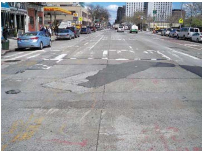
Figure 13.10. An example of city street pavement with many utility cuts (First Avenue, New York City). Source: The Fort Miller Co., Inc.
