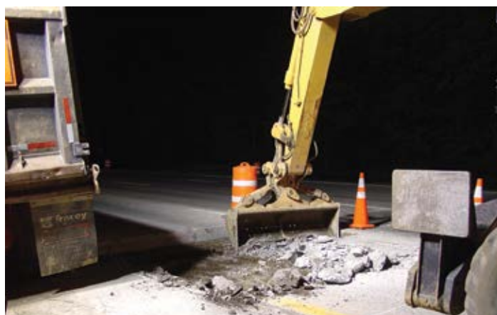
Figure 8.24. The shattered pavement seen here had to be removed with an excavator even though the lift-out method was specified. Source: The Fort Miller Co., Inc.
