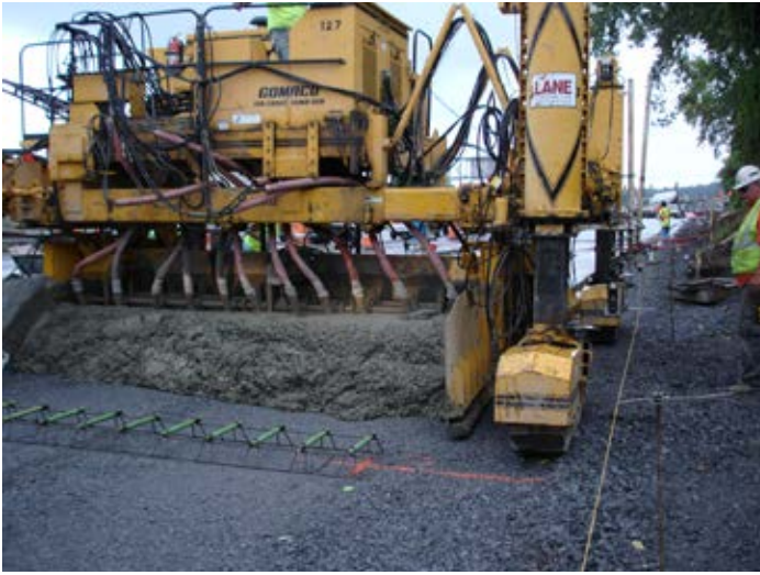
Figure 1.3. String line controlled slip-form paver approaching dowel basket (note vibrators for consolidation). Source: The Fort Miller Co., Inc.
