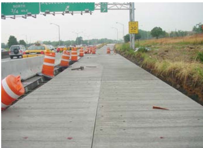
Figure 4.4. Wide precast concrete ramp pavement in Long Island, N.Y., with a longitudinal joint in the center of the lane. Source: The Fort Miller Co., Inc.
