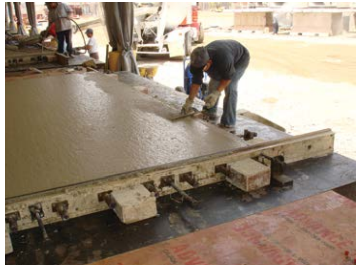
Figure 7.22. Worker touching up the screeded surface near the side rails. Source: The Fort Miller Co., Inc.
