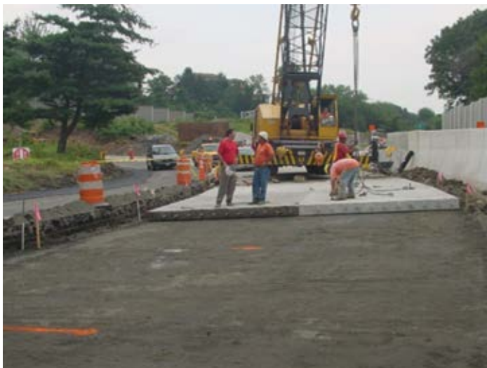
Figure 8.15. Panel points, identified with red paint, being used on a PCP project. Source: The Fort Miller Co., Inc.
