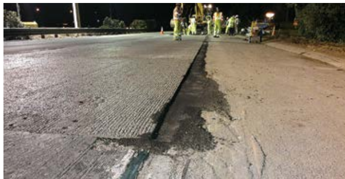
Figure 11.37. This new asphalt – placed directly against new precast panels – was barely wide enough to allow proper and uniform compaction. Source: The Fort Miller Co., Inc.
