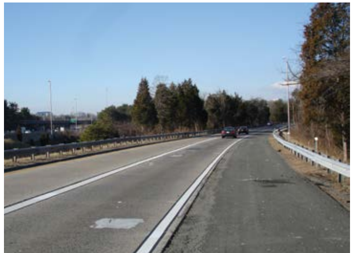
Figure 3.11. The right-hand lane of a high-speed exit ramp in Fairfax, Va., that was replaced during overnight full ramp closures. Source: The Fort Miller Co., Inc.
