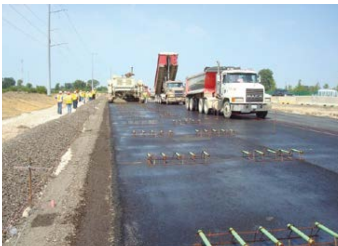
Figure 4.22. 2013 photos of conventional paving and precast repairs using only wheel path dowels on Illinois Tollway projects. Source: Pavement Engineering and Research Consultants, LLC
