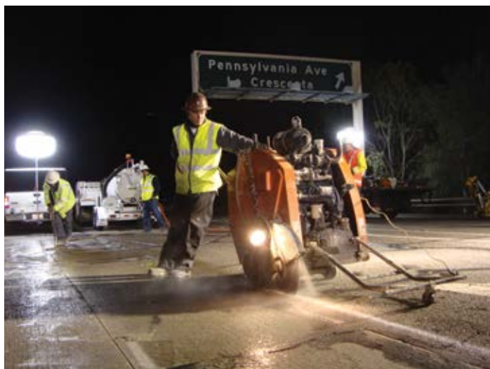
Figure 8.17. This sawing crew is equipped with adequately sized saws, proper lighting, a water supply and a slurry suction truck. Source: The Fort Miller Co., Inc.
