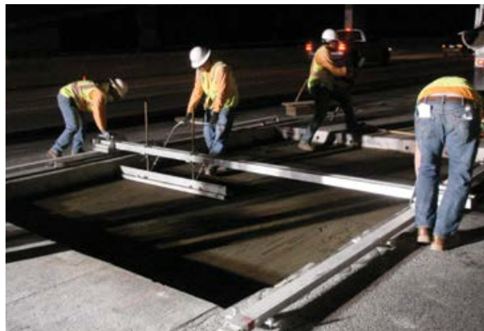
Figure 10.13. A four-man crew grading fine aggregate bedding material. Source: The Fort Miller Co., Inc.
