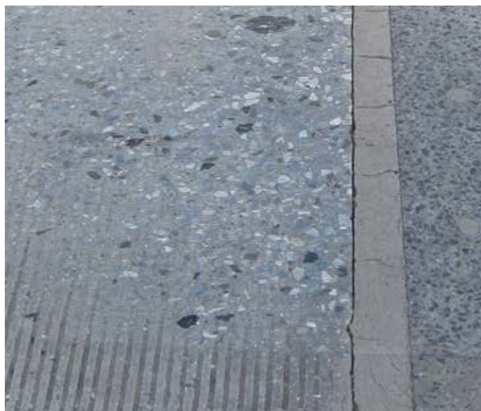
Figure 12.6. Hairline cracks in a wide-grouted joint, an indicator of possible early grout material failure. Source: The Fort Miller Co., Inc.
