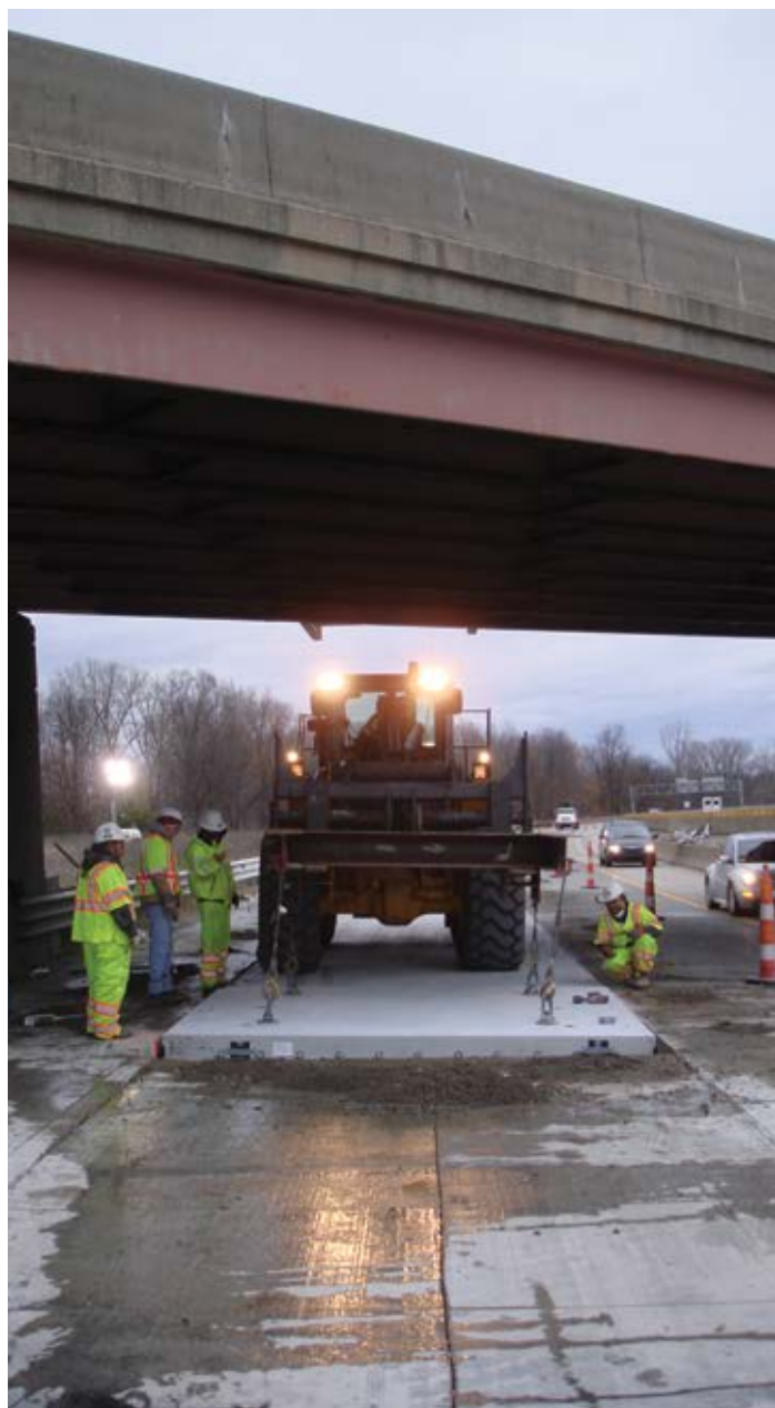
Figure 5.6 Example of a one-lane work area provided to replace the same lane. Source: The Fort Miller Co., Inc.
