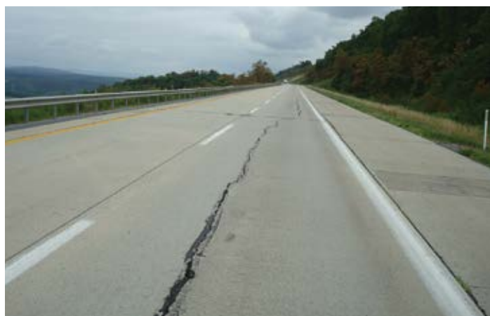
Figure 2.10: Longitudinal crack (possibly due to foundation support issues). Source: Pavement Engineering and Research Consultants, LLC
