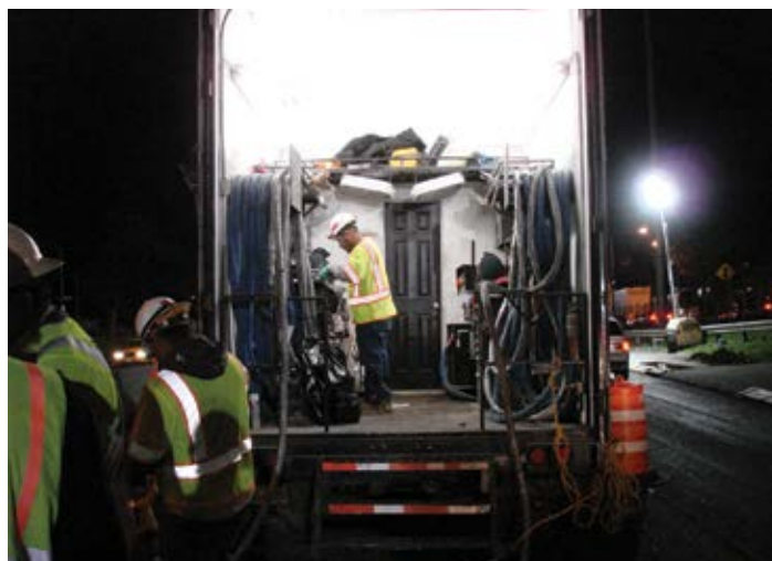
Figure 9.20. A fully equipped urethane injection support truck. Source: The Fort Miller Co., Inc.
