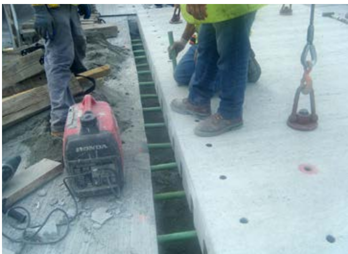
Figure 11.11. The over-width transverse joint in this photo was likely caused by incorrect layout of the end saw cut in the existing pavement on the left. Source: The Fort Miller Co., Inc.
