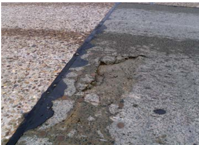
Figure 11.15. This photo shows a Super-Slab panel that shattered around the dowels in the adjacent precast panel after it was grouted. Source: The Fort Miller Co., Inc.
