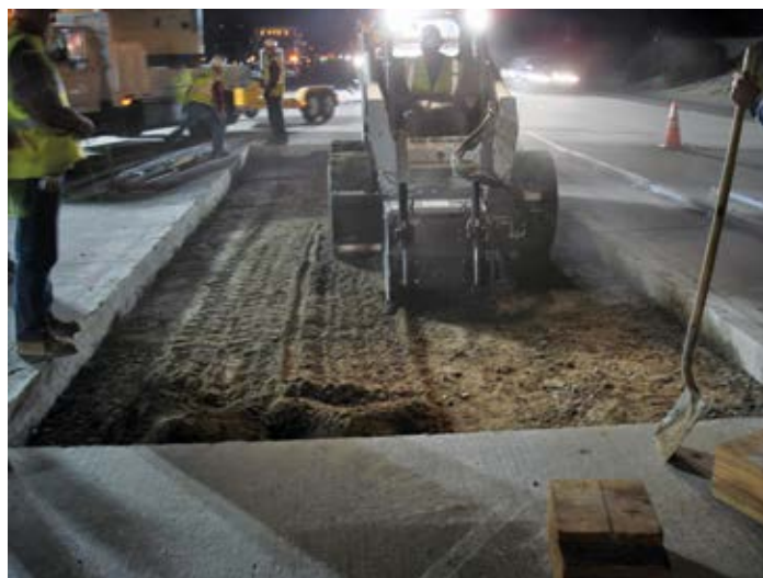
Figure 2.15. Removal of cement-treated base using a skid-steer-mounted milling machine on Interstate 210 in Tarzana, Calif. Source: The Fort Miller Co., Inc.
