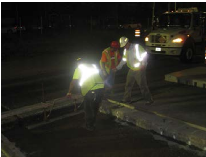
Figure 10.19. A representative of a grade-supported PCP system trains a screed operator. Source: The Fort Miller Co., Inc.
