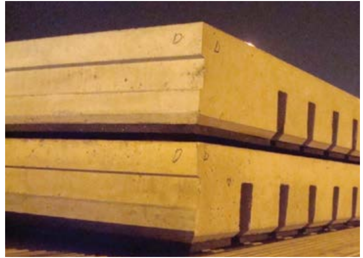
Figure 4.18. Keyways on longitudinal joints of precast pavement panels. Source: M.B. Snyder, Pavement Engineering and Research Consultants, LLC
