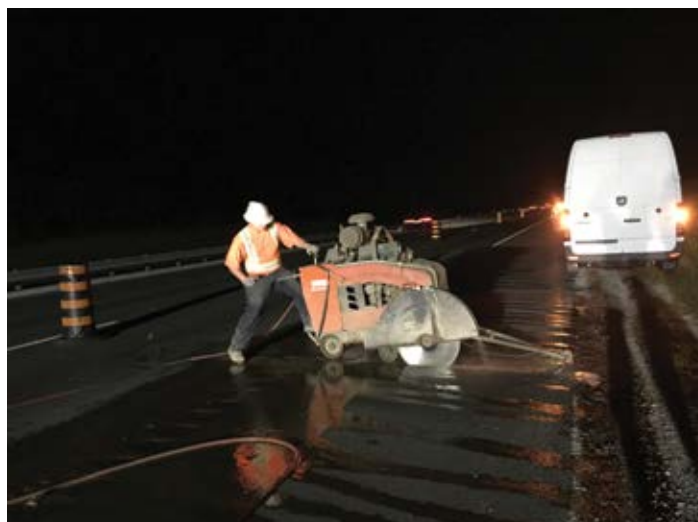
Figure 13.14. A transverse saw cut being made at the terminus of a single night's installation. Source: The Fort Miller Co., Inc.
