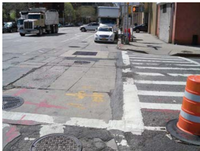
Figure 2.17. Urban intersection requiring repair with numerous utility access points. Source: The Fort Miller Co., Inc.
