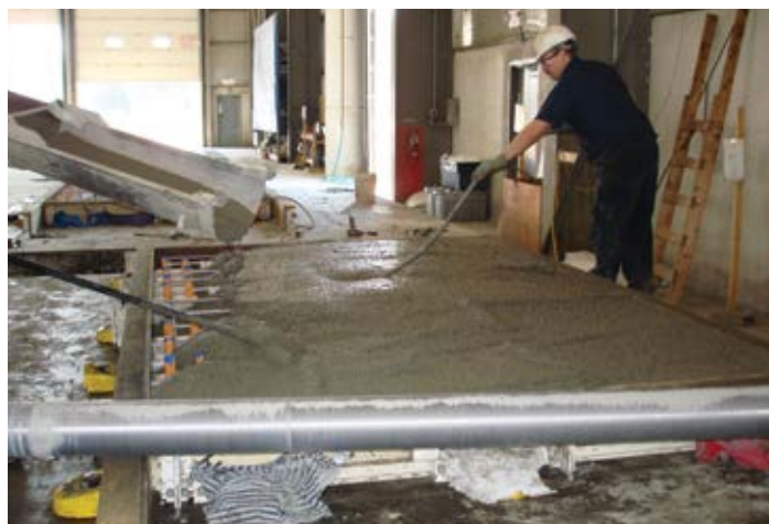
Figure 7.20. Concrete placement directly from a ready-mix truck (form is low enough to permit direct placement from the truck). Source: The Fort Miller Co., Inc.
