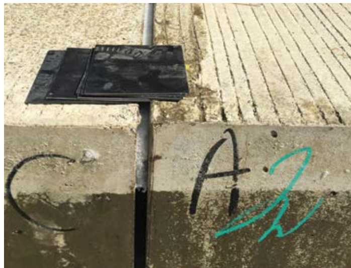
Figure 10.9. Two shims left behind indicate an actual vertical differential of 1/8 inch between the two panels. Source: The Fort Miller Co., Inc.
