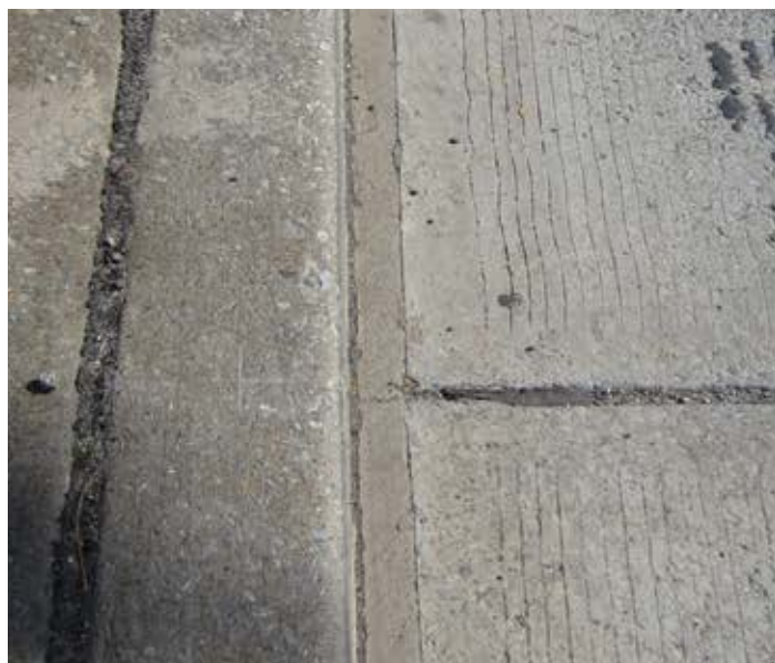
Figure 12.7. This 1.5-inch-wide, grout-filled longitudinal joint, located between an existing curb on the left and precast panels on the right, is performing well after being in service for more than five years. Source: The Fort Miller Co., Inc.
