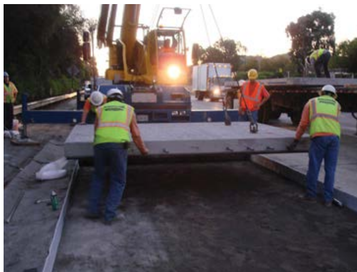
Figure 10.16. An ideally sized panel placement crew of five, with one man in each corner and one man on the truck. Source: The Fort Miller Co., Inc.
