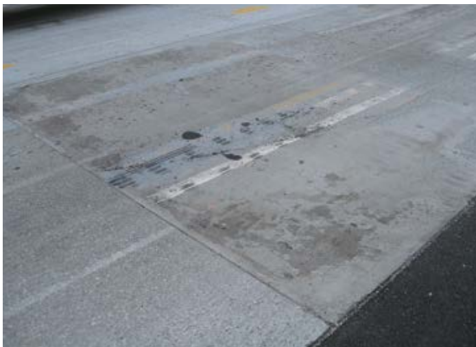
Figure 11.23. Non-uniform surface texture produced by partial coverage by diamond grinding machine. Source: The Fort Miller Co., Inc.
