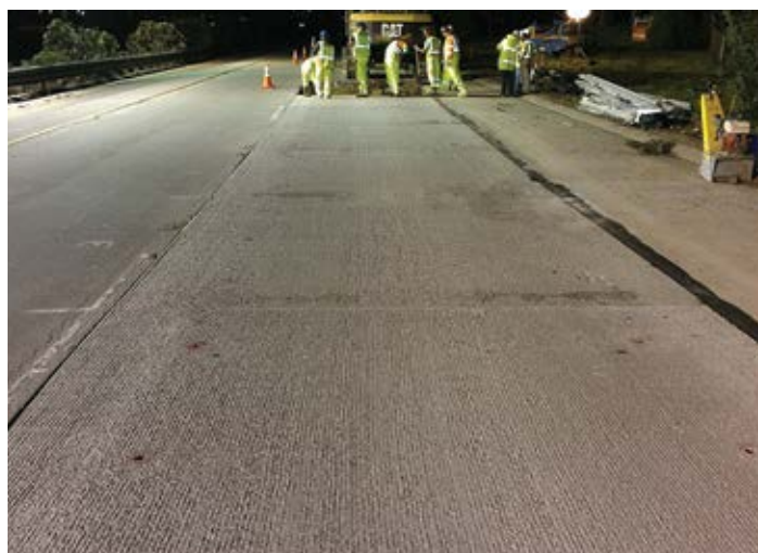
Figure 3.7. Example use of multiple JPrCP panels in a single repair. Source: The Fort Miller Co., Inc.
