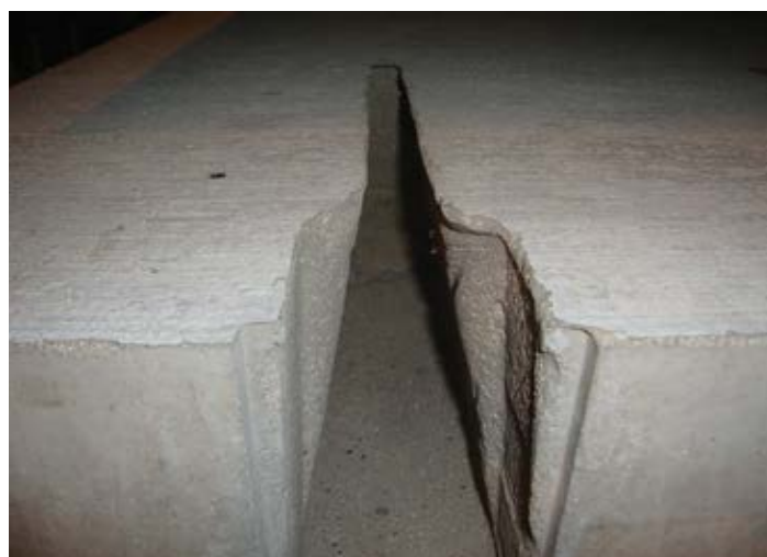
Figure 9.33. Slot openings in the Illinois Tollway system are dovetail in shape (narrower at the top than at the bottom). Source: Performance Plus Products, LLC
