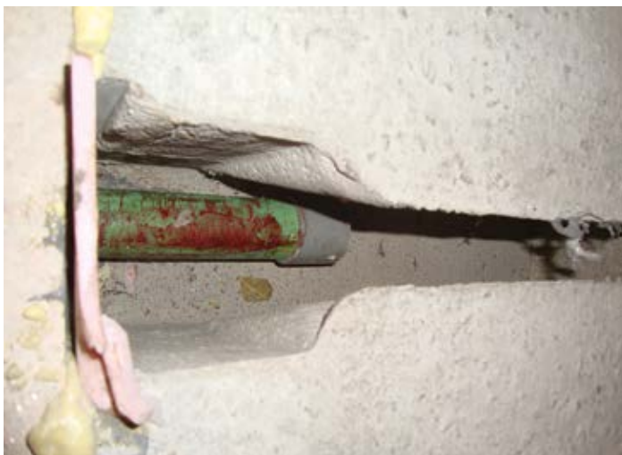
Figure 9.34. The hole drilled for the dowel in this photo was not closely aligned with the cast-in slot, making dowel installation difficult. Source: Performance Plus Products, LLC
