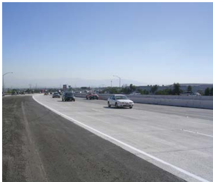
Figure 12.1. Interstate 15 in Ontario, Calif., carries approximately 200,000 vehicles per day and includes high-quality precast panels (seen in the left two lanes) that were installed in a series of eight-hour night work windows. Source: Pro-Cast Products
