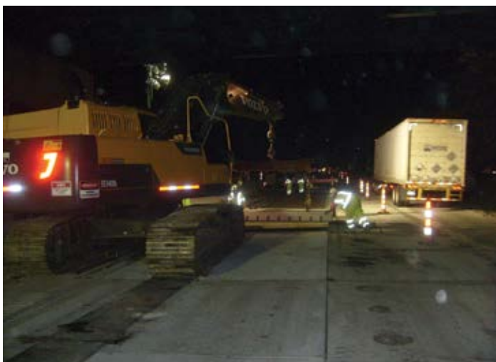
Figure 9.50. A track-mounted excavator placing a PCP panel under an overpass on Interstate 94 in Kalamazoo, Mich. Source: The Fort Miller Co., Inc.
