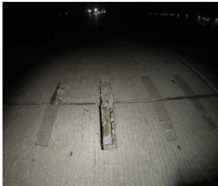
Figure 12.4. Bond failure between the grout encasing the dowel and the vertical sides of the slot. Source: Performance Plus Products, LLC
