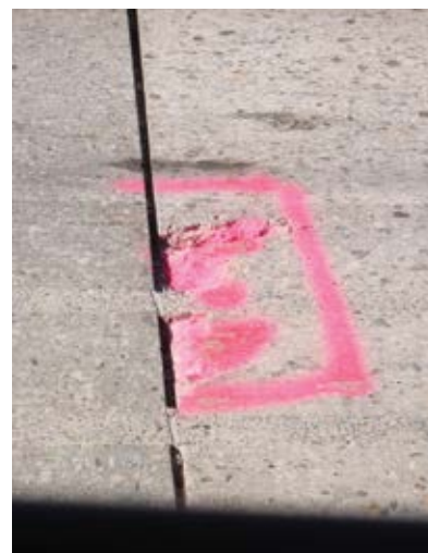
Figure 11.4. Photo showing failure of backfill material in top slots around the dowels and failure of the concrete between the slots. Source: The Fort Miller Co., Inc.
