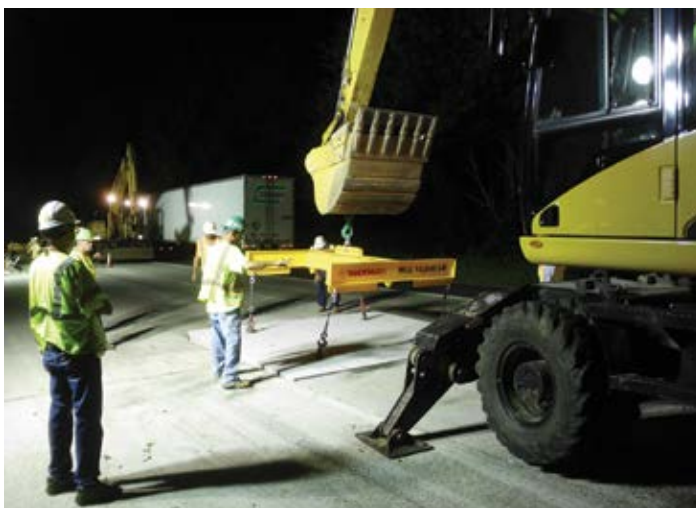
Figure 9.47. The outrigger of this rubber-tired excavator is located outside of the PCP panel area. Source: The Fort Miller Co., Inc.
