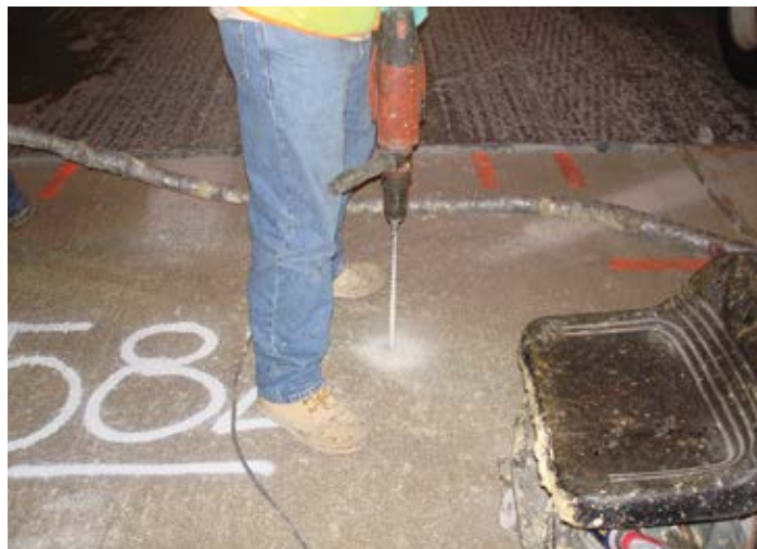
Figure 9.12. A worker drills a new foam port in a part of the panel that needs extra force to provide vertical uplift. Source: The Fort Miller Co., Inc.
