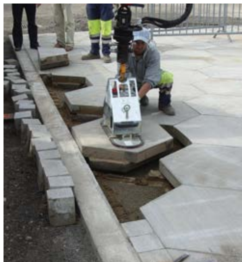
Figure 13.11. Hexagonal removable urban pavement system installed in Nantes, France. Source: Laboratoire Central des Ponts et Chaussées
