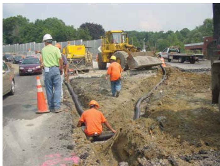
Figure 8.30. Extensive subbase repair prior to JPrCP installation (visible in the background). Source: The Fort Miller Co., Inc.
