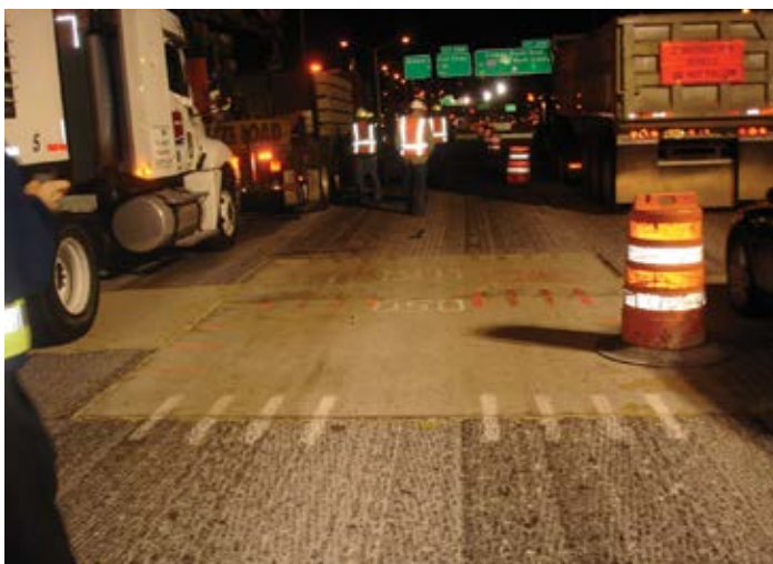
Figure 9.21. Two newly installed panels marked out for field saw cutting at precast-to-precast and precast-to-existing joints. Source: The Fort Miller Co., Inc.
