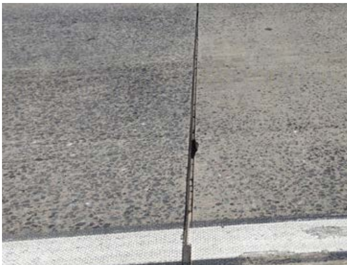
Figure 12.8. Joint-filling grout between the silicone seal on the left and the panel on the right has de-bonded from the panel, creating a maintenance problem in this variable-width joint. Source: The Fort Miller Co., Inc.
