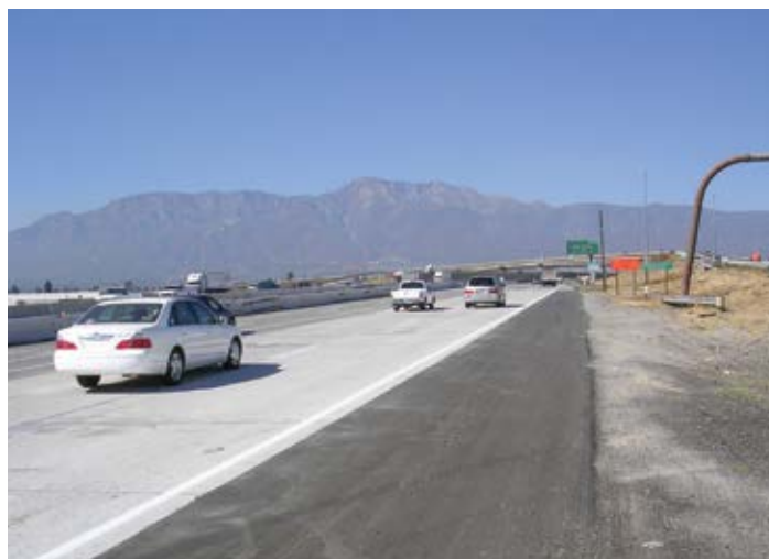
Figure 3.8. Tangent lane replacement of a portion of Interstate 15 near Ontario, Calif., using JPrCP. Source: The Fort Miller Co., Inc.
