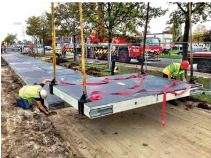
Figure 13.27. Precast power-generating panels being installed on accurately graded bedding material. Source: Laboratoire Central des Ponts et Chaussées
