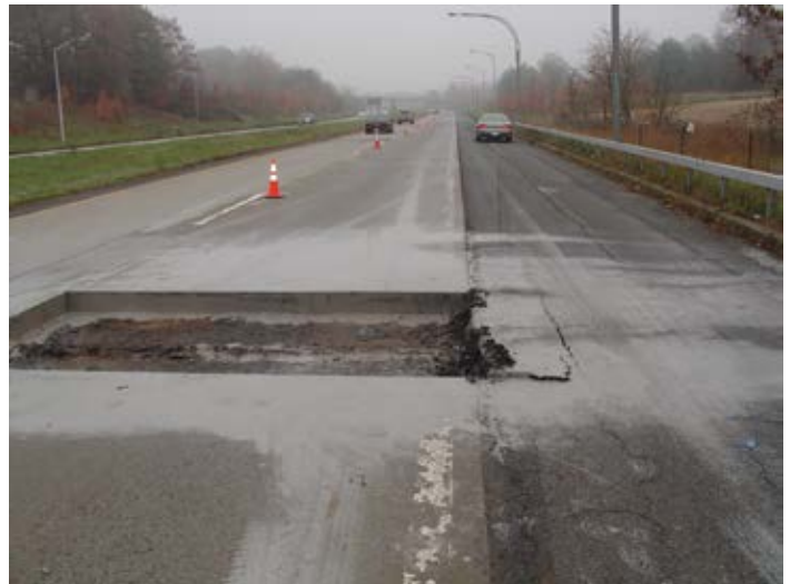
Figure 8.14. Failure to cut the asphalt shoulder prior to pavement removal resulted in serious shoulder damage on this project. Source: The Fort Miller Co., Inc.
