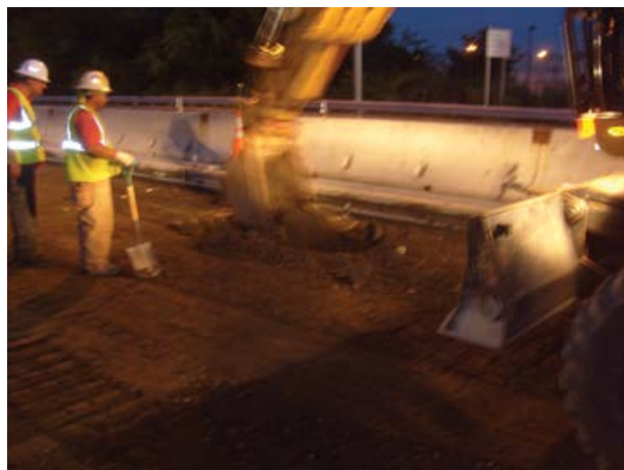
Figure 8.29. Spot repair during subbase preparation. Source: The Fort Miller Co., Inc.
