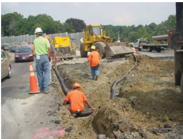
Figure 2.16. Installation of pavement drainage prior to the use of PCP panels. Source: The Fort Miller Co., Inc.
