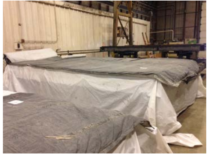
Figure 7.25. A newly casted panel covered with plastic and insulating blankets for initial curing. Source: The Fort Miller Co., Inc.
