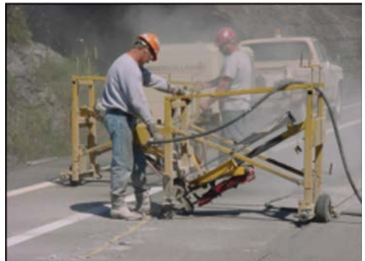
Figure 9.40. A worker uses a pneumatic drill to create cross-stitch holes across a longitudinal slab crack. Source: National Concrete Pavement Technology Center
