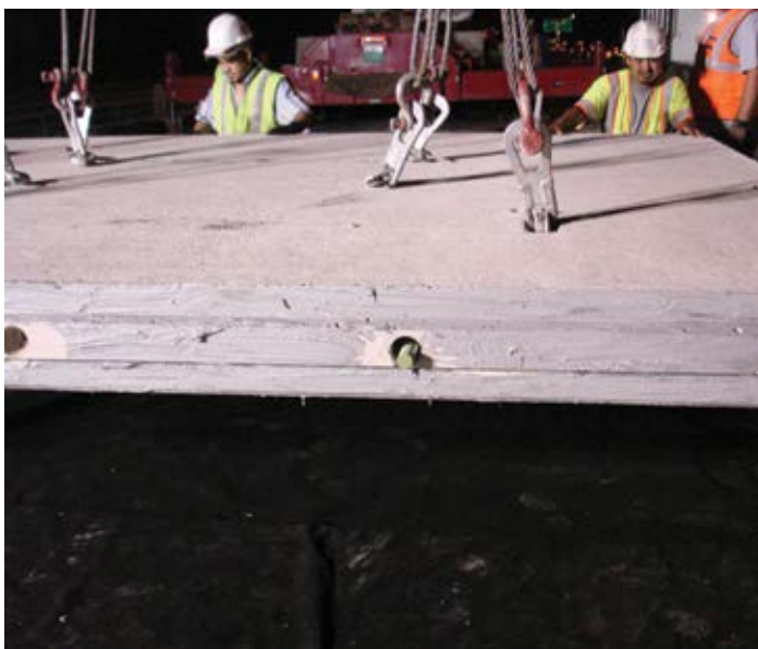
Figure 12.12. SwiftLift lifting inserts are favored by some precasters because they allow quick and safe attachment of lifting cables to precast panels. Source: The Fort Miller Co., Inc.
