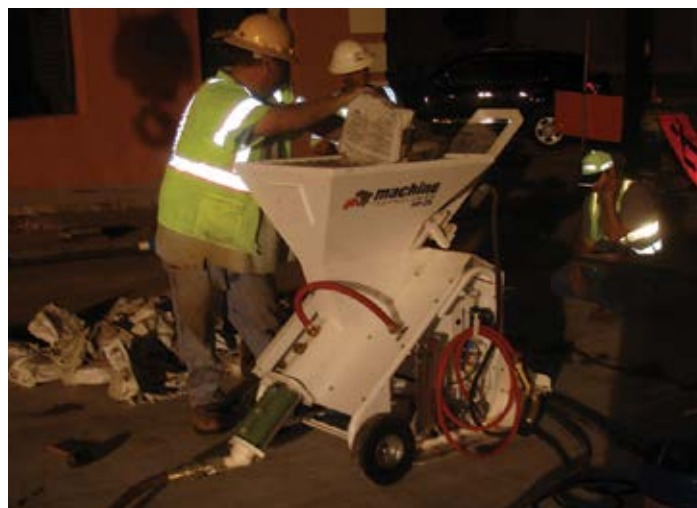
Figure 9.16. Workers dumping grout powder into the top of a volumetric mixer/pump. Source: The Fort Miller Co., Inc.
