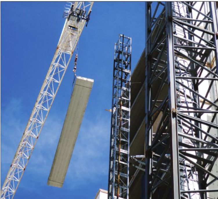
This worker is completing an installation of hollow-core slab.
