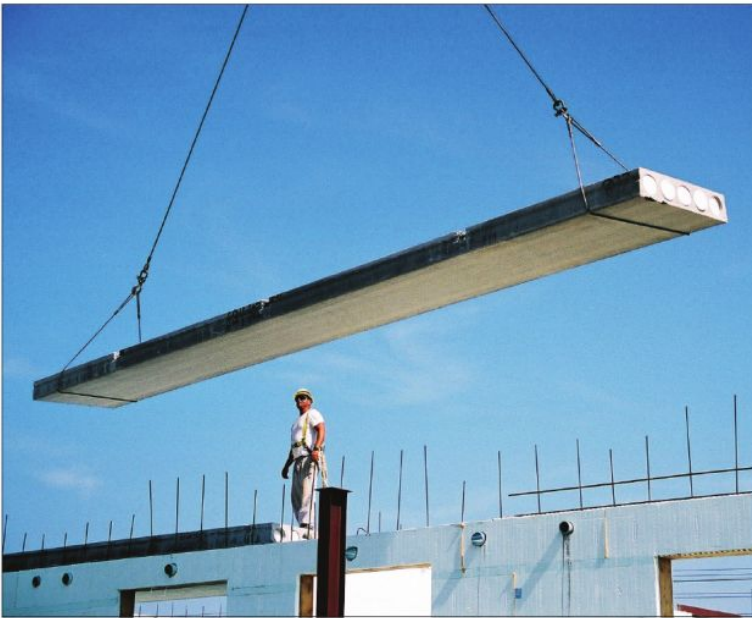
This worker is completing an installation of hollow-core slab.
